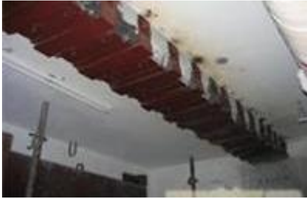
Figure 3. Steel jacking retrofit of a beam in a building
