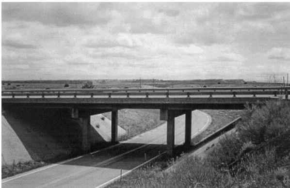
Figure 1. A typical high way bridge in US
