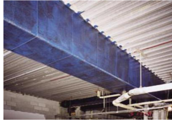
Figure 4. Picture showing beam retrofit using CFRP
