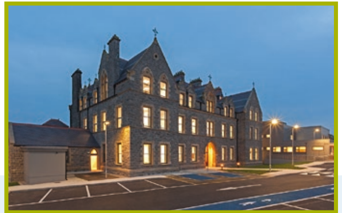
▲ Ballyshannon Primary Care Centre
