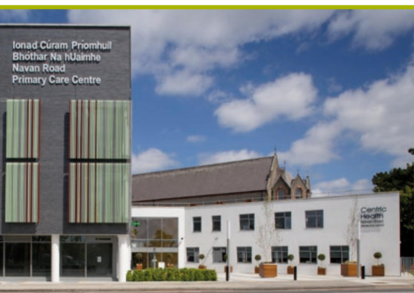
▲ Navan Road Primary Care Centre (Photo: Paul Tierney)
