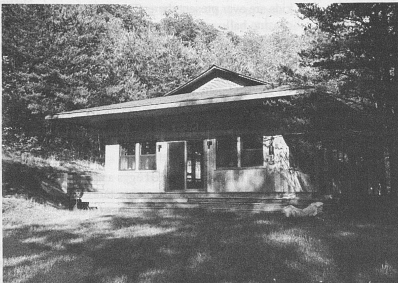
Furnace Zen Center Dharma Room near Lexington, Kentucky.
