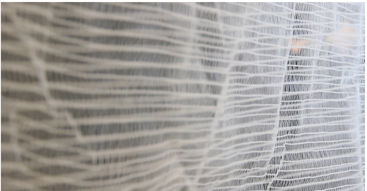
Fig. 3.22 Detail of textile prototype. Video still from competition entry with Vivienne La and Freya Robinson. Facing page: fig. 3.23 Plan of AJ6 showing relationship of distorted frames to the layered glazing of the Design Hub façade.
