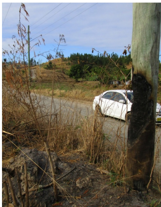
Figure 2. Infrastructure damage due to fire. Photo: Robert Harrison
