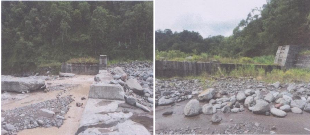
Gambar 17. Sabo Dam KD-4
