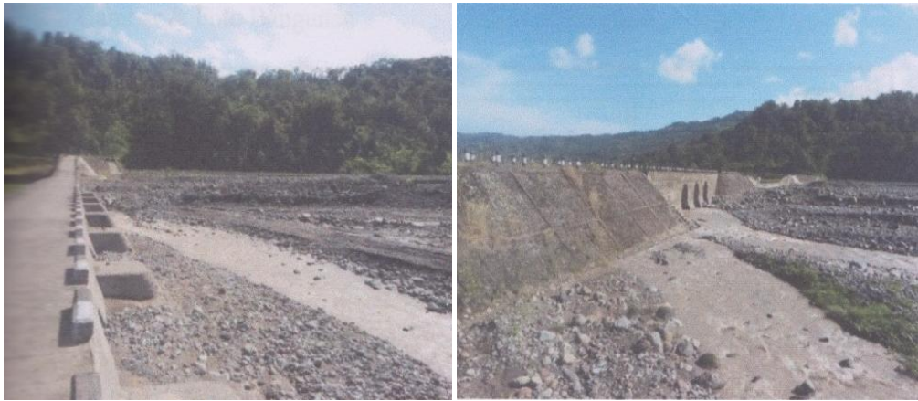
Gambar 12. Sabo Dam KD-1
