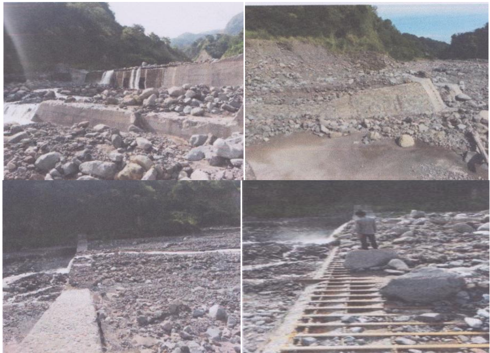
Gambar 4. Sabo Dam No. 7-4
