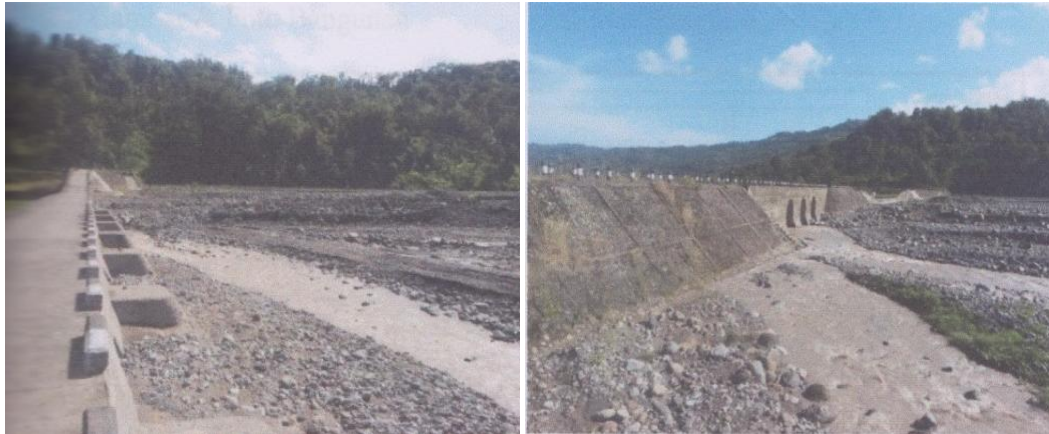
Gambar 2.12 Consolidation Dam Bili-bili ( Sumber : Konsultan PT. Aria, 2014 )
