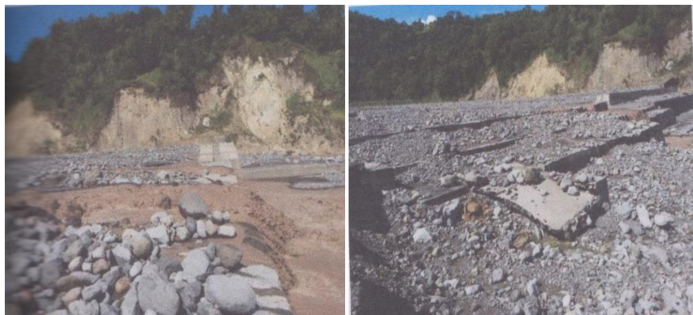
Gambar 16. Sabo Dam KD.3
