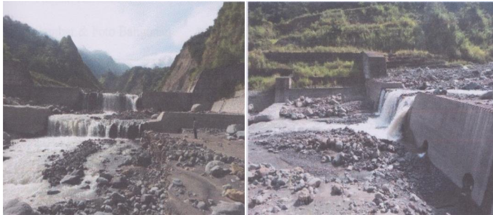
Gambar 5. Sabo Dam No. 7-5
