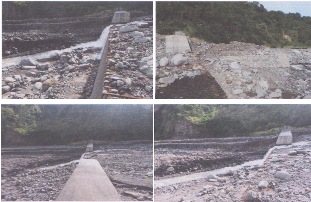
Gambar 3. Sabo Dam No. 7-3
