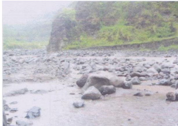
Gambar 8. Sabo Dam CD-1
