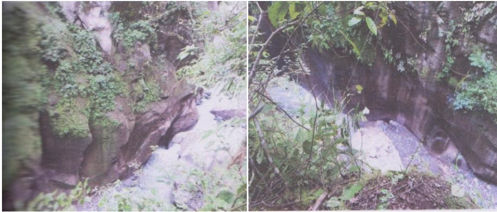
Gambar 11. Sabo Dam CD-4
