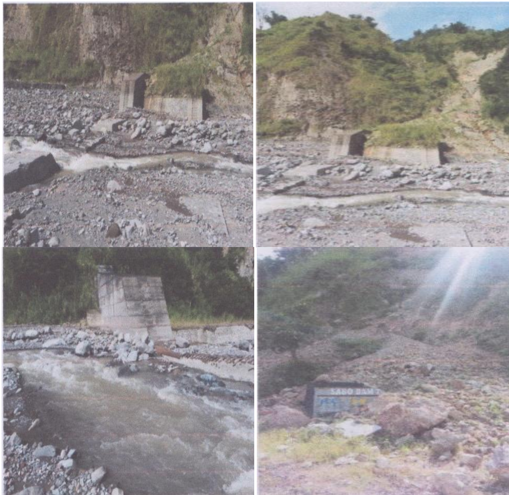
Gambar 6. Sabo Dam No. 7-6
