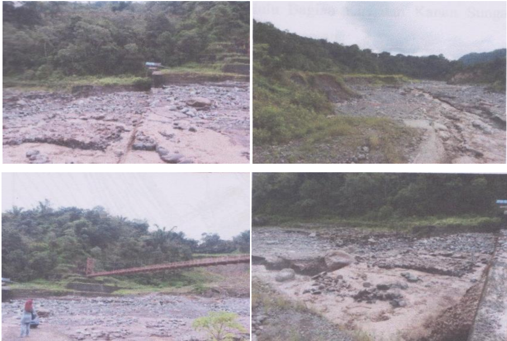
Gambar 9. Sabo Dam CD-2
