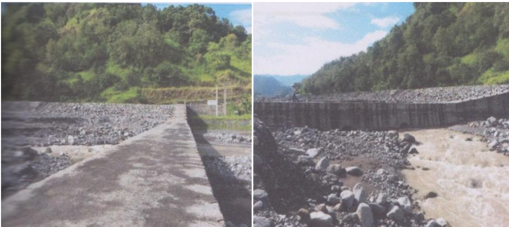
Gambar 13. Sabo Dam KD-2
