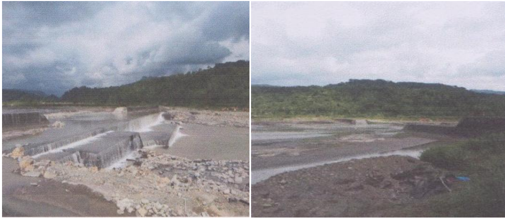
Gambar 18. Sabo Dam SP-1
