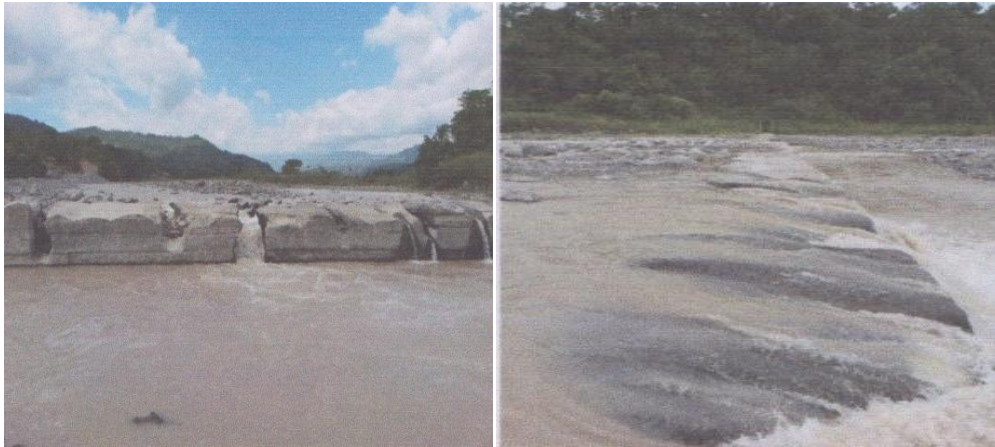
Gambar 20. Sabo Dam SP-3
