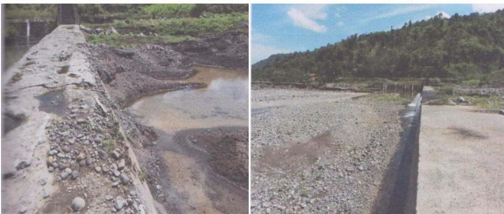
Gambar 22. Sabo Dam SP-5
