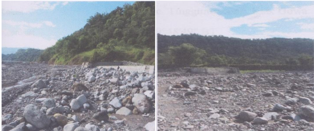
Gambar 14. Sabo Dam KD.2-1
