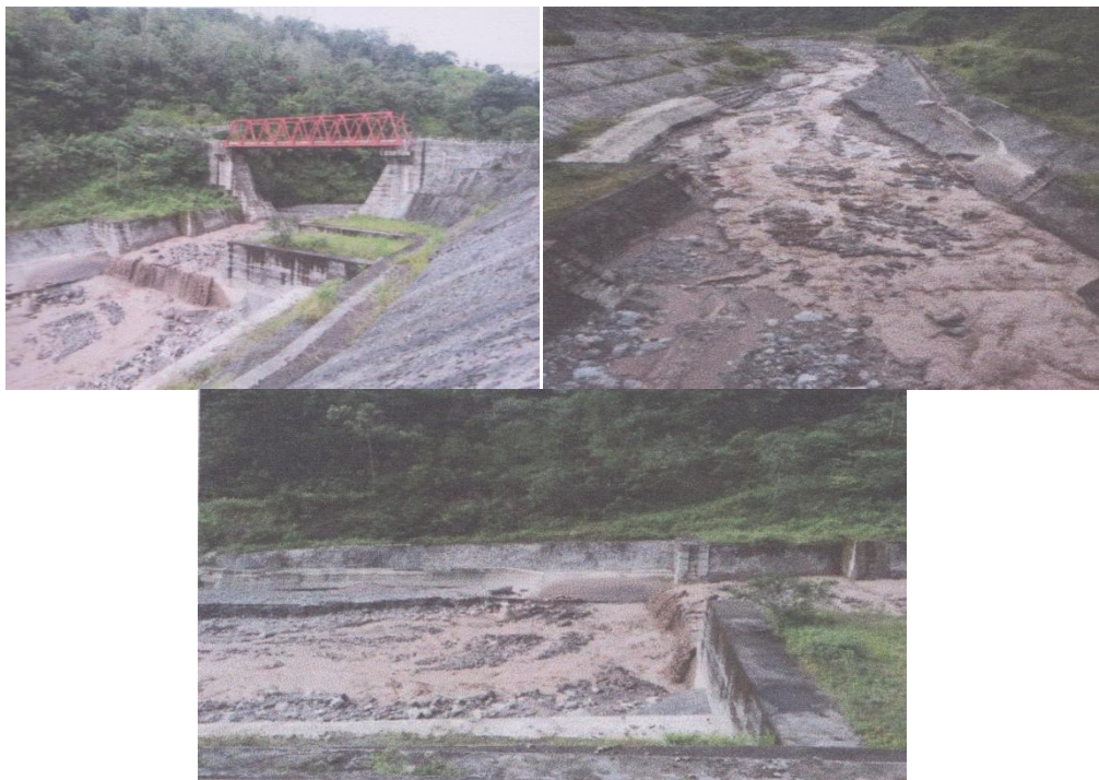
Gambar 10. Sabo Dam CD-3
