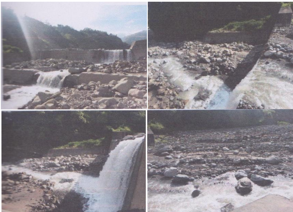
Gambar 2. Sabo Dam No. 7-2
