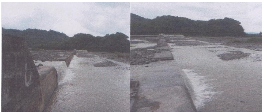
Gambar 19. Sabo Dam SP-2
