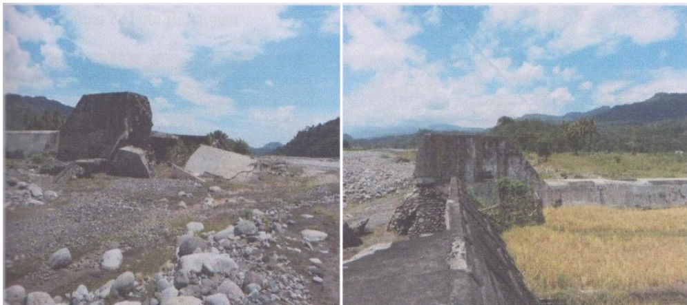
Gambar 21. Sabo Dam SP-4
