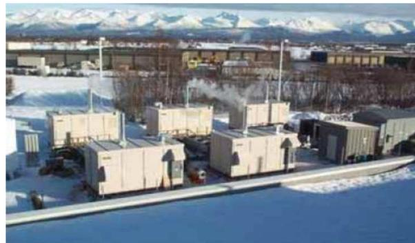
FIG. IV-23 – CENTRALE DES PILES À COMBUSTIBLE EN ALASKA DE 1 MW DE PUISSANCE [GON 2004]
