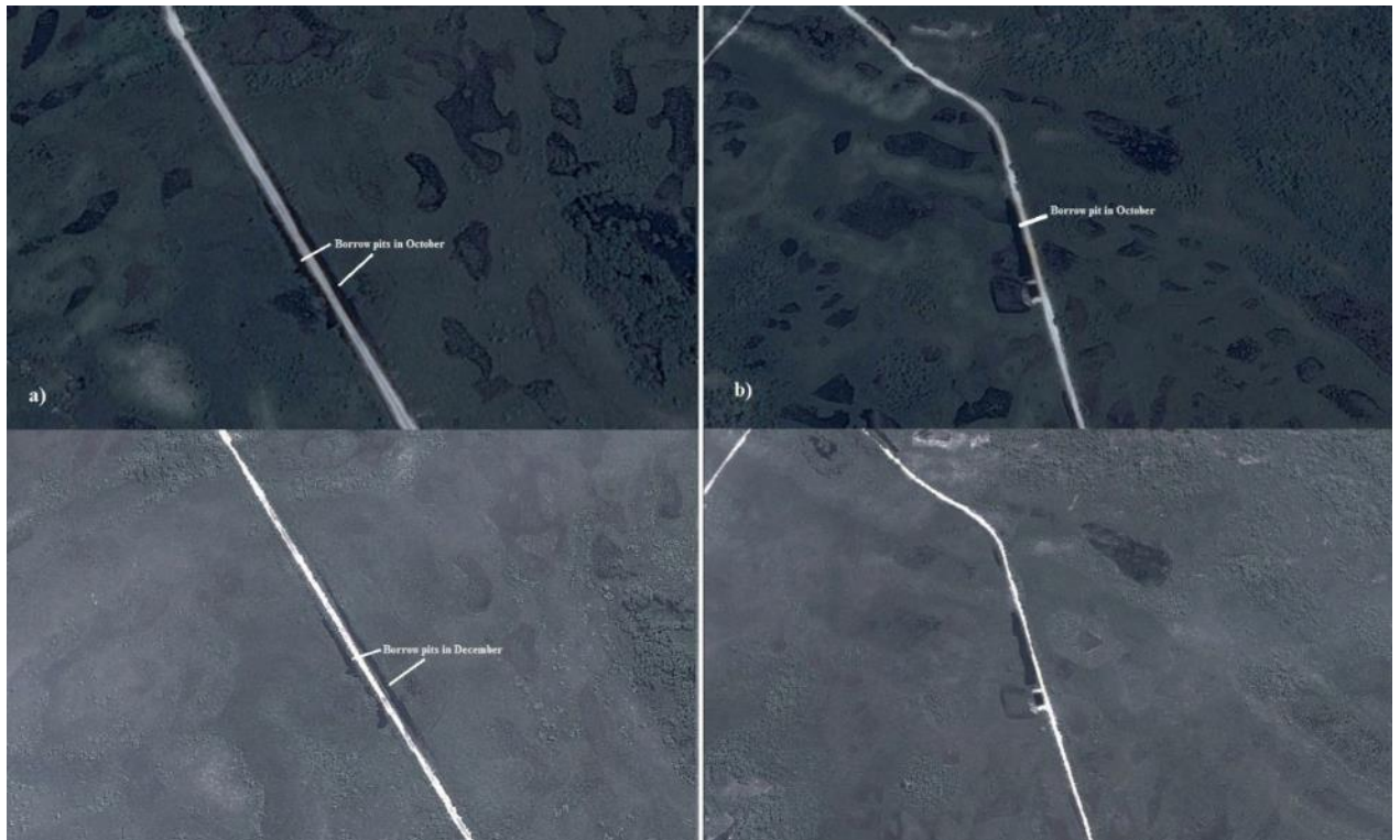
Figure 4.2. Aerial views of sites along Chesapeake Rd south of Northcliffe. a) Two borrow pits surrounded by inundated wetland in October (Google earth V 7.1.2.2041, 24 October, 2013a) and again in December with the surrounding wetland dry (Google earth V 7.1.2.2041, 27 December, 2011a), b) A single borrow pit also surrounded by inundated wetlands in October (Google earth V 7.1.2.2041, 24 October, 2013b), and again still inundated when the surrounding wetland is dry in December (Google earth V 7.1.2.2041, 27 December, 2011b)
