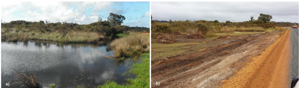
Figure 4.1. Western most Fouracres Rd site surveyed in a) winter, note the dirt road on the top right, b) when visited after summer, clearly showing the site has been lost due to road widening, note the construction vehicle still in the image along with the road in the process of becoming bituminised
