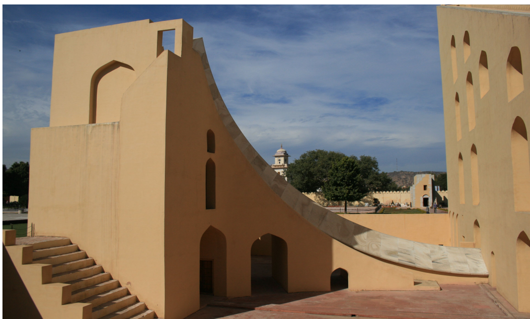
A view of the Samrat Yantra at Jaipur: The instrument enables celestial measurements to be taken relating to the equator and the world's axis. The large semi-circle forms a plan parallel to the equator, while the triangular structure points to the celestial plane, forming a line parallel to the world's axis.
