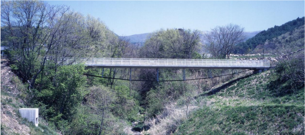
Figure 8: Tobu recreation resort footbridge (courtesy of Meguru Tsunomoto, Oriental Construction Co)
