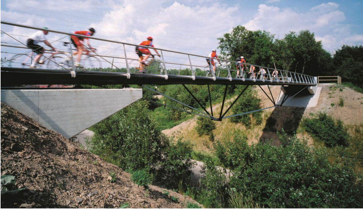
Figure 7: Jumet footbridge (courtesy of Jean Marie Cremer, Bureau Greisch)
