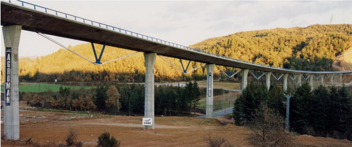
Figure 6: Osormort viaduct (courtesy of Javier Manterola, Carlos Fernández Casado S.L.)
