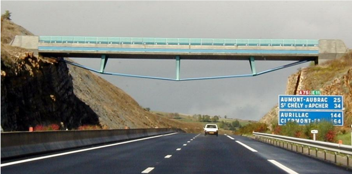
Figure 5: Truc de la Fare overpass (courtesy of Nicolas Janberg, www.structurae.de )
