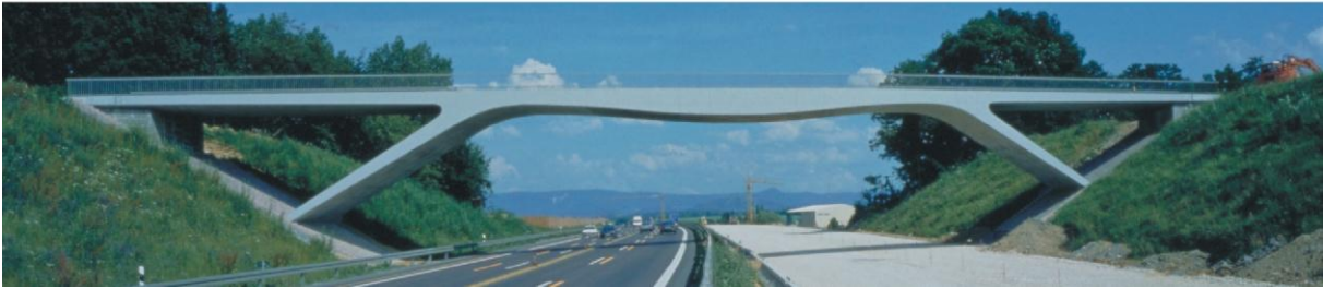
Figure 3: Kirchheim overpass, (a) proposal (courtesy of Jörg Schlaich, ©Schlaich, Bergermann und Partner)and (b) built structure (courtesy of Jörg Schlaich, ©Elsner Gert, Stuttgart)
