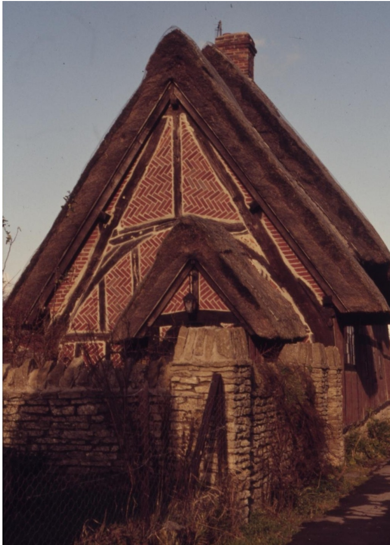
Fig. 8. A smoke-bay house: Pomander Cottage, Harwell, Oxon: (a) end view showing thatch layering and (b) side view. The smoke-bay is marked by posts on either side of the inserted left-hand chimney (photographs 1970, 1986) (CC).
