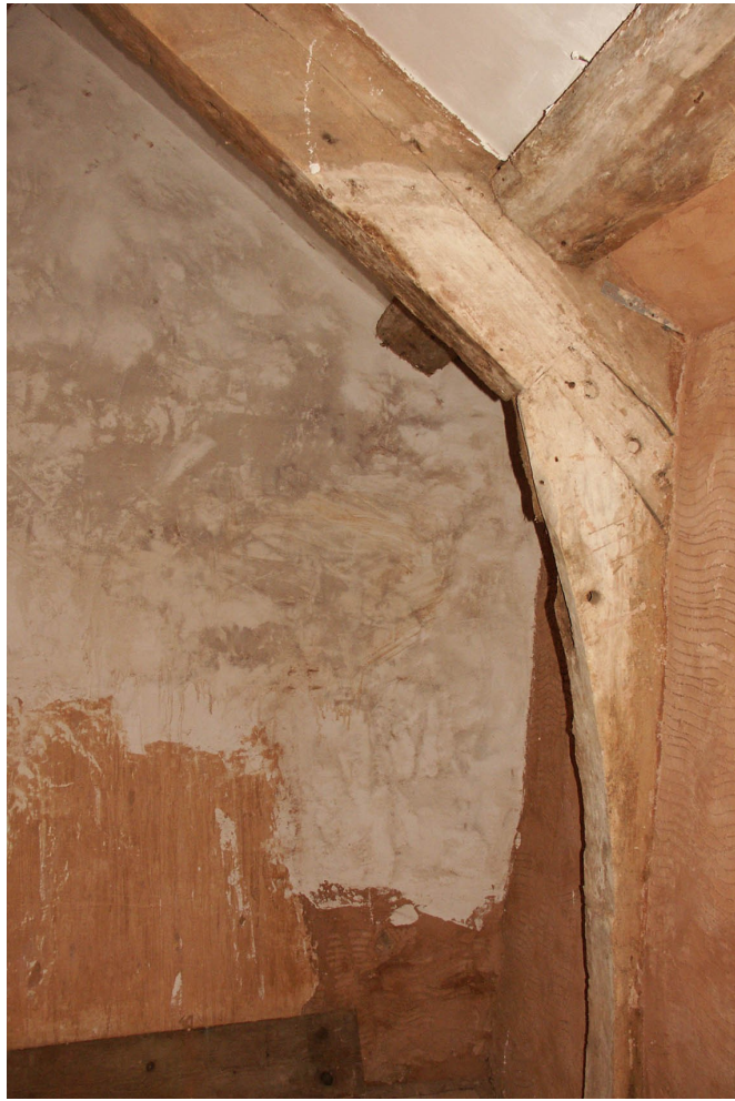
Fig. 13. Jointed-cruck trusses: a) Clerks, Spaxton, Somerset; b) comparative section drawings (NWA).
