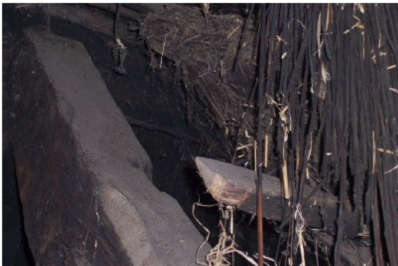
Fig. 7. Sooted rafter, lath, thatch, under-thatch: Hill, Christow, Devon, 2008 (CC).
