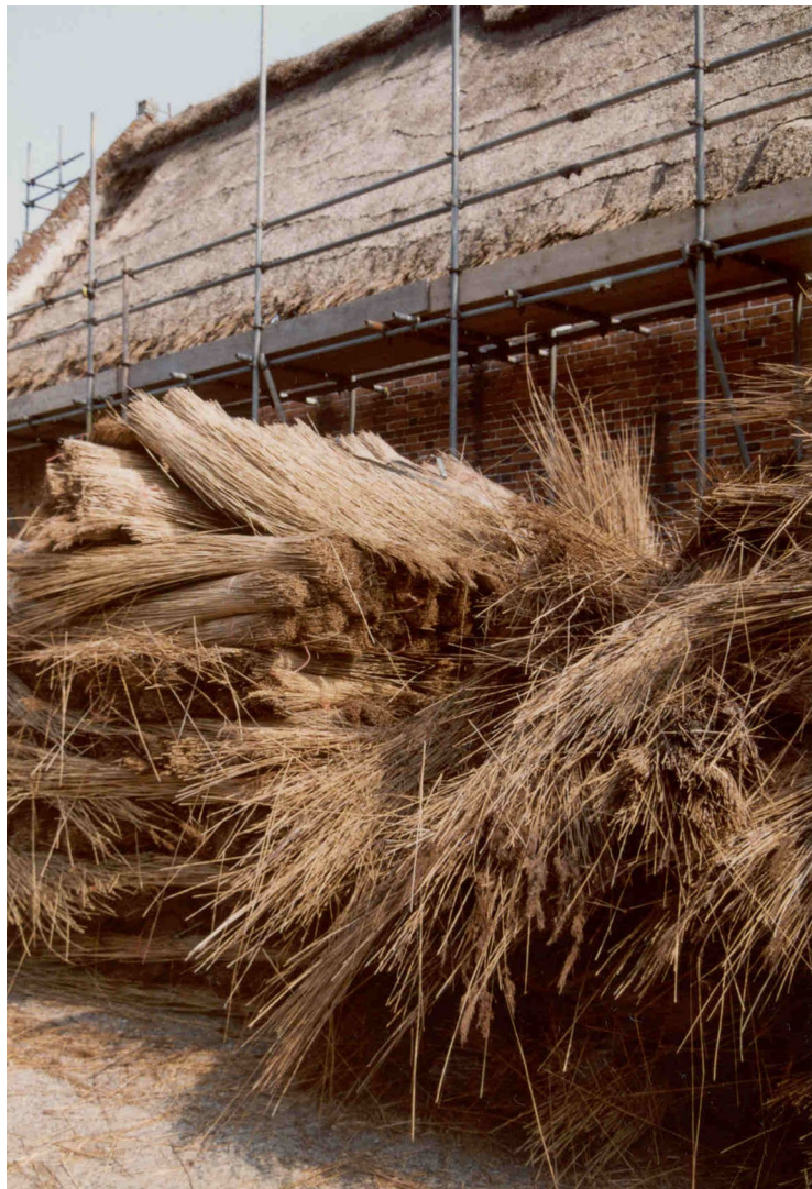
Fig. 2 Water-reed thatch: (a) Waxham barn, Norfolk; (b) thatching at Catfield, Norfolk (both NWA).
