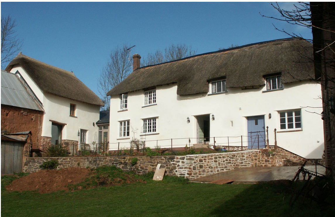
Fig. 4. Combed-straw thatching: Elley, Colebrooke, Devon (NWA).
