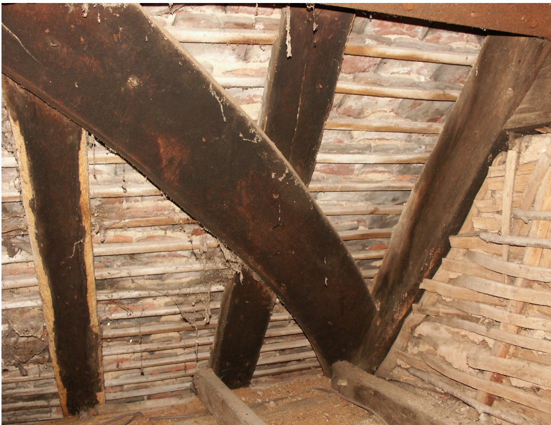
Fig. 6. Sooted roof-timbers: Old Rectory, Clifford Chambers, Warwickshire (NWA).
