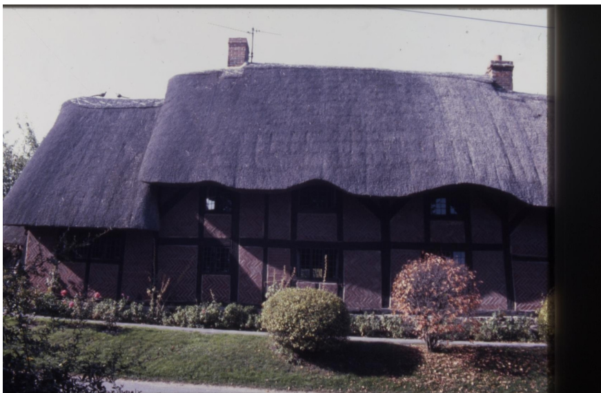
Fig. 8. A smoke-bay house: Pomander Cottage, Harwell, Oxon: (a) end view showing thatch layering and (b) side view. The smoke-bay is marked by posts on either side of the inserted left-hand chimney (photographs 1970, 1986) (CC).
