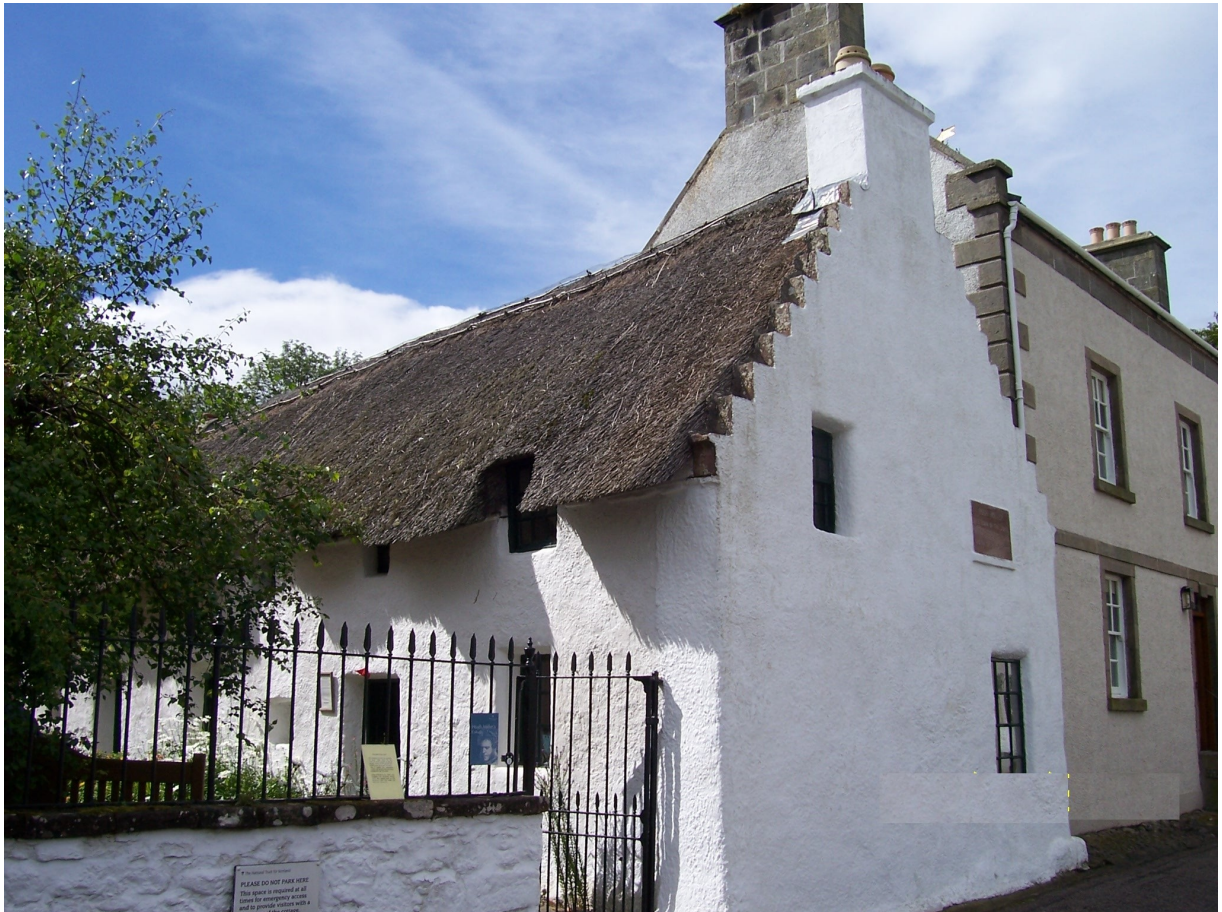
Fig. 1. Mixed thatch with heather – Hugh Miller's Cottage, Cromarty, Scotland: (a) general view; (b) detail (CC).
