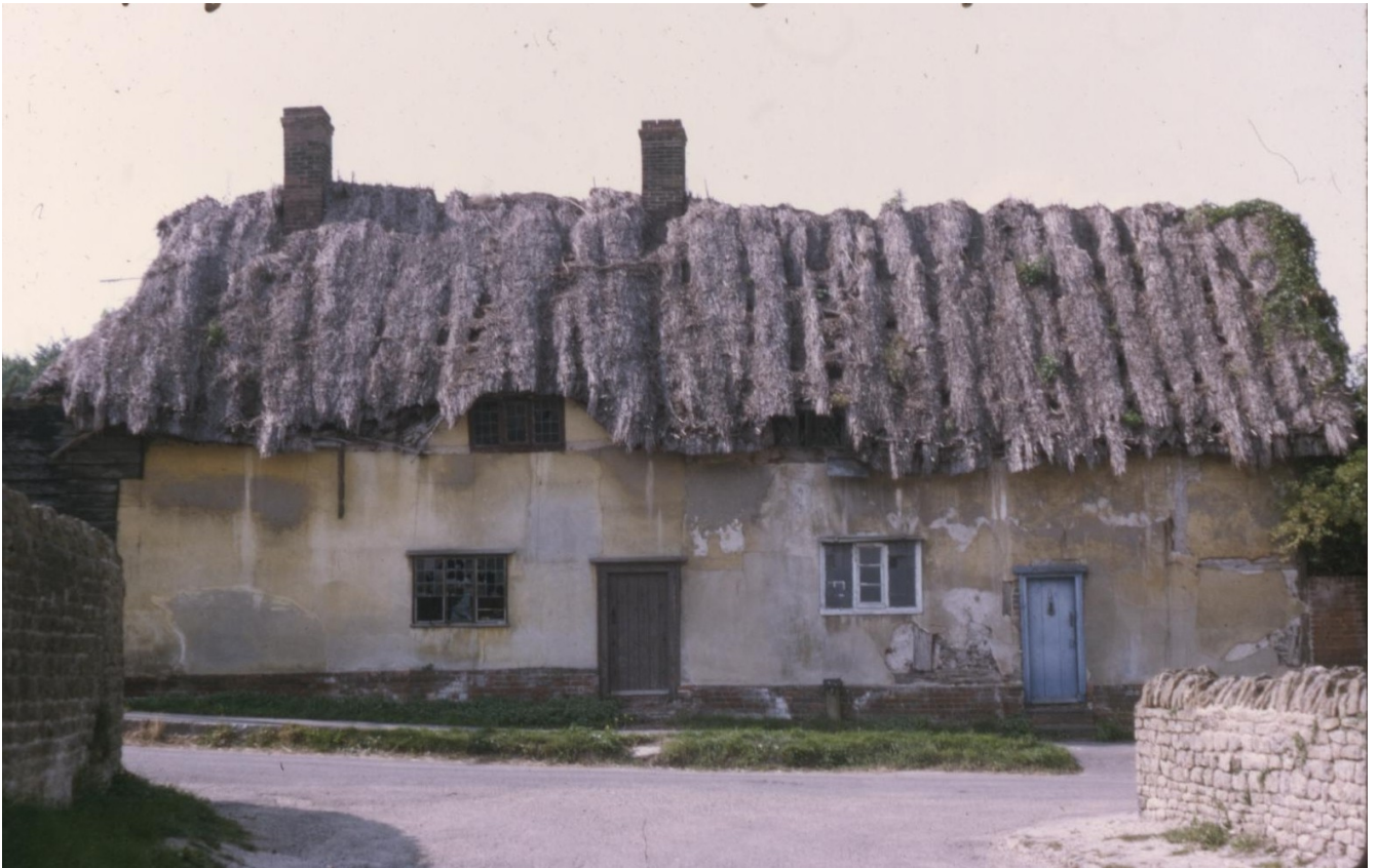
Fig. 3. Very decayed long-straw thatch in 1971: Godfrey's Farm, East Hendred, Oxon.[then Berks.] (CC).
