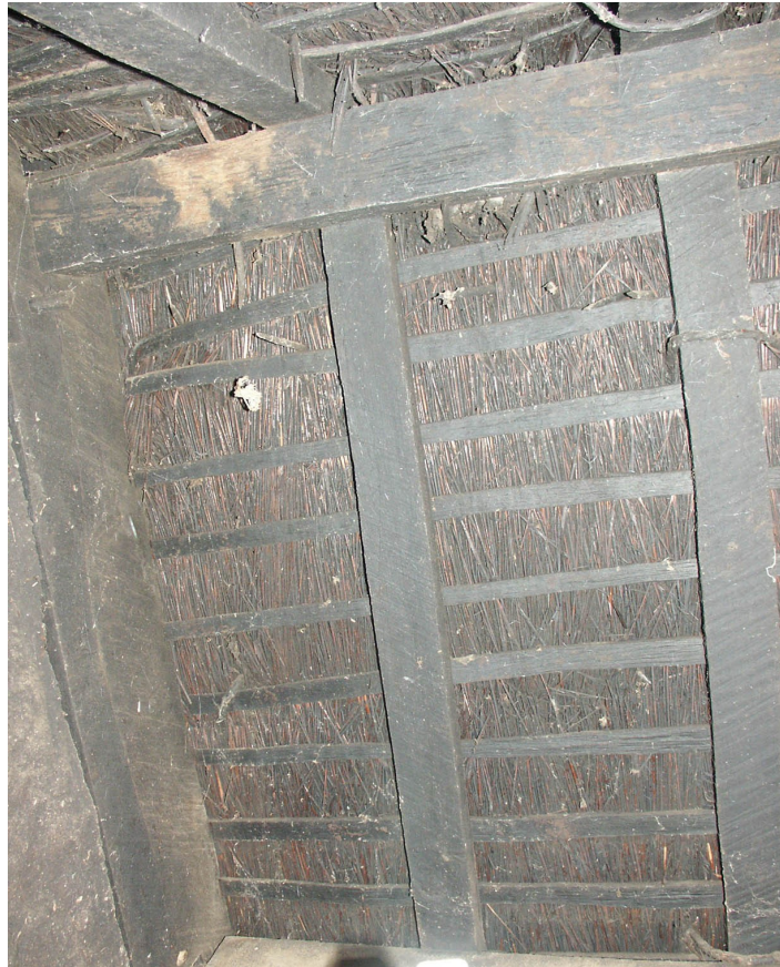
Fig. 17. Lower Chilverton, Coldridge, Devon: interior of roof showing thatch (NWA).
