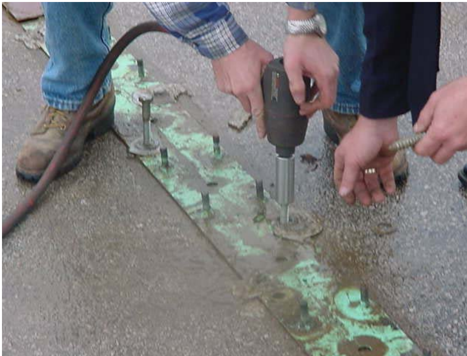
Figure B3. Lag Bolt and Anchor Plate Removal.
