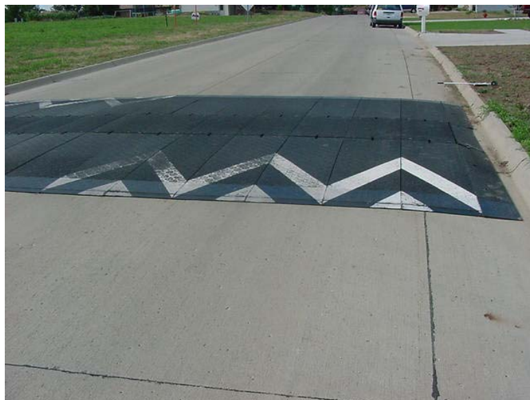
Figure 23. Pavement Markings on Speed Hump/Table
