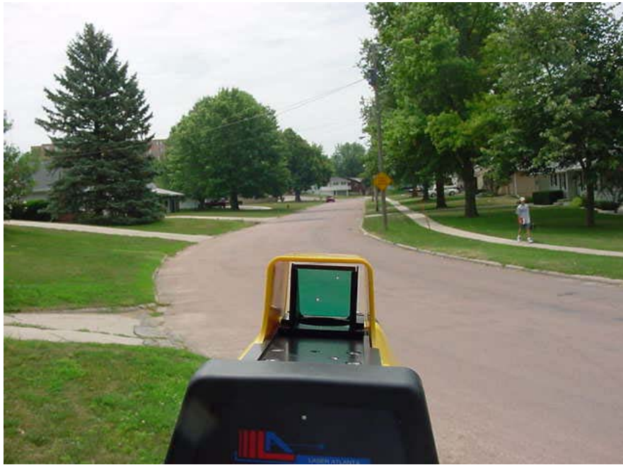
Figure 27. Southbound Data Collection View on Roosevelt Drive
