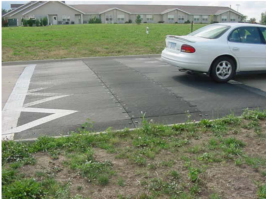
Figure 18. 18-Foot Temporary 30 mph Speed Table
