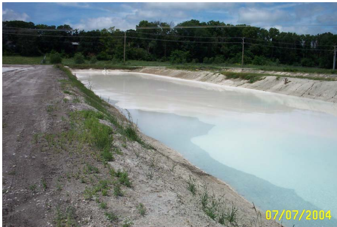
Figure 1: Dewatering Lagoon While Filling
