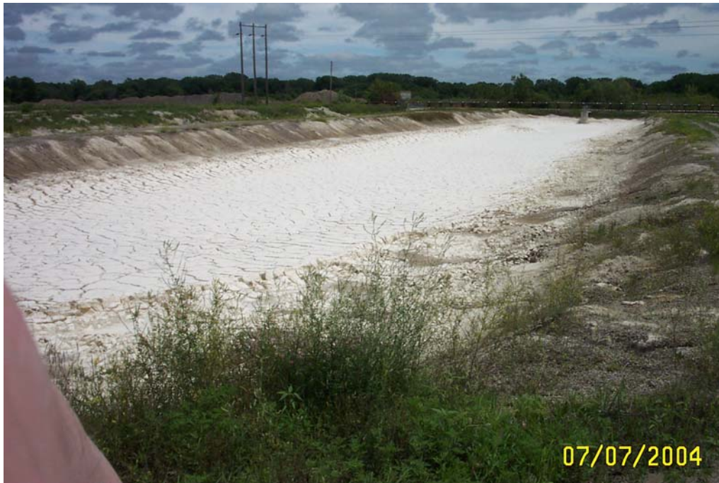
Figure 3: Dewatering Lagoon after 10 Months Settling
