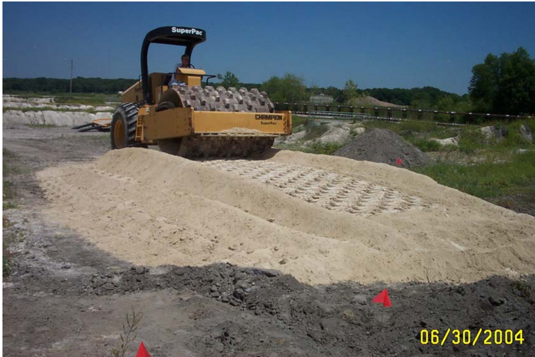
Figure 60: Compacting the test embankment
