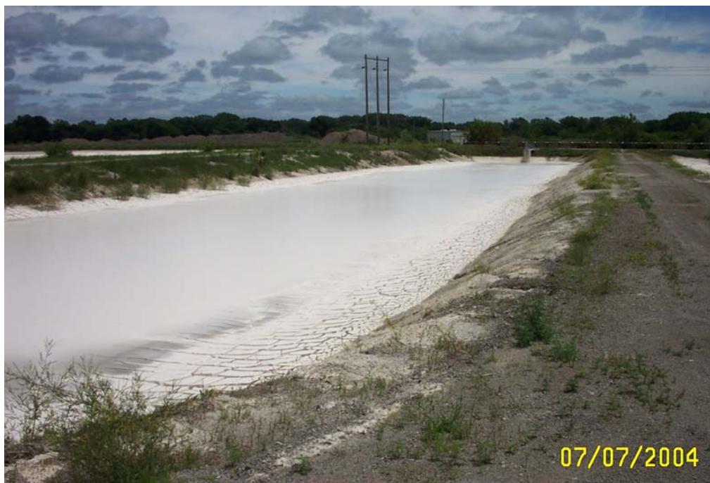
Figure 2: Dewatering Lagoon after 3 Months Storage
