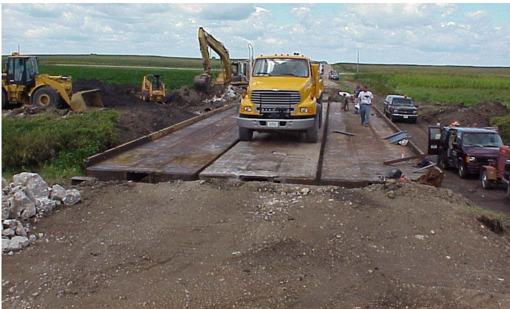
Figure 4.22. Field load testing the unconnected RRFCs during WCB LT1.
