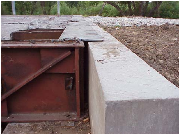
f. Expansion joint at the west abutment
