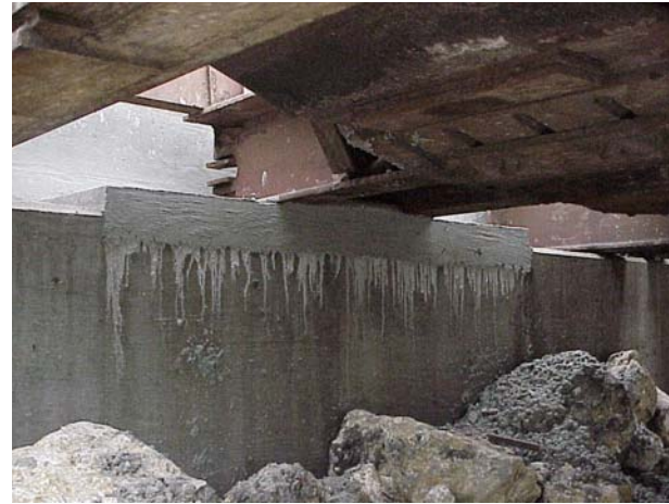
e. Completed interior girder seat
