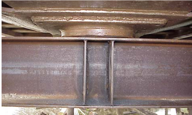
e. Web stiffeners under the bolster at the piers
