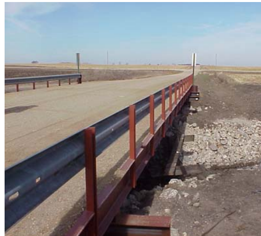
b. Installation of the thrie beam
