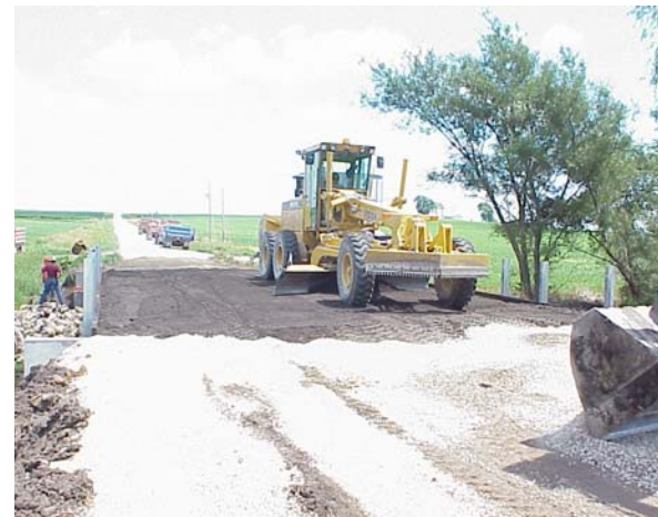
d. Blading the asphalt milling driving surface
