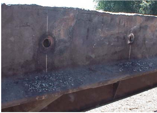
a. Drilled holes for the transverse threaded rod
