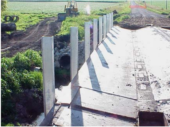
a. Guardrail posts welded on the BCB
