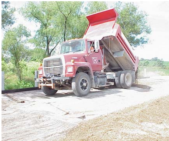
c. Laying pea gravel
