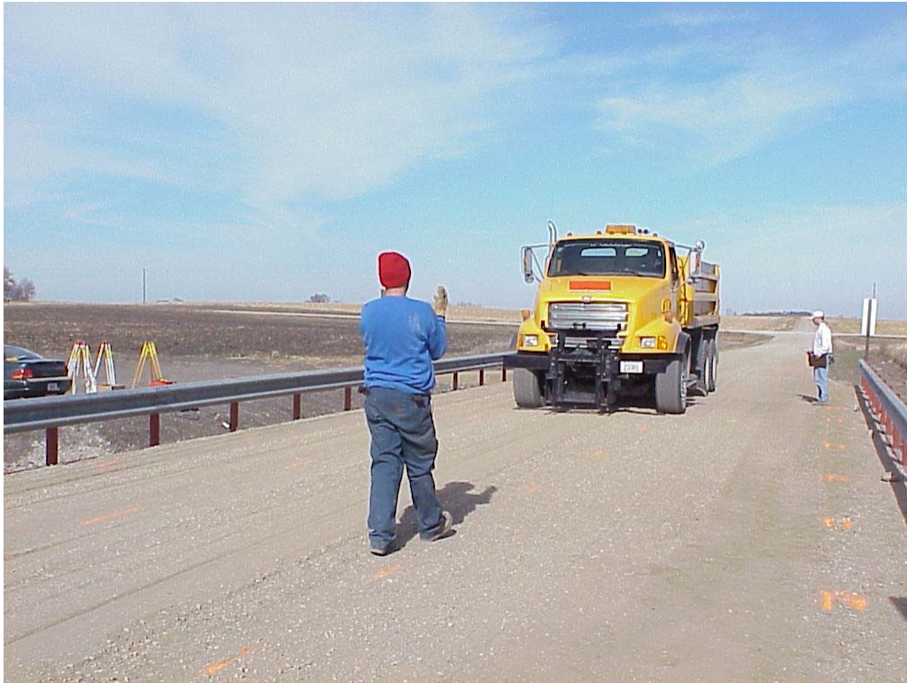
Figure 4.25. Testing the finished WCB immediately following completion of construction.
