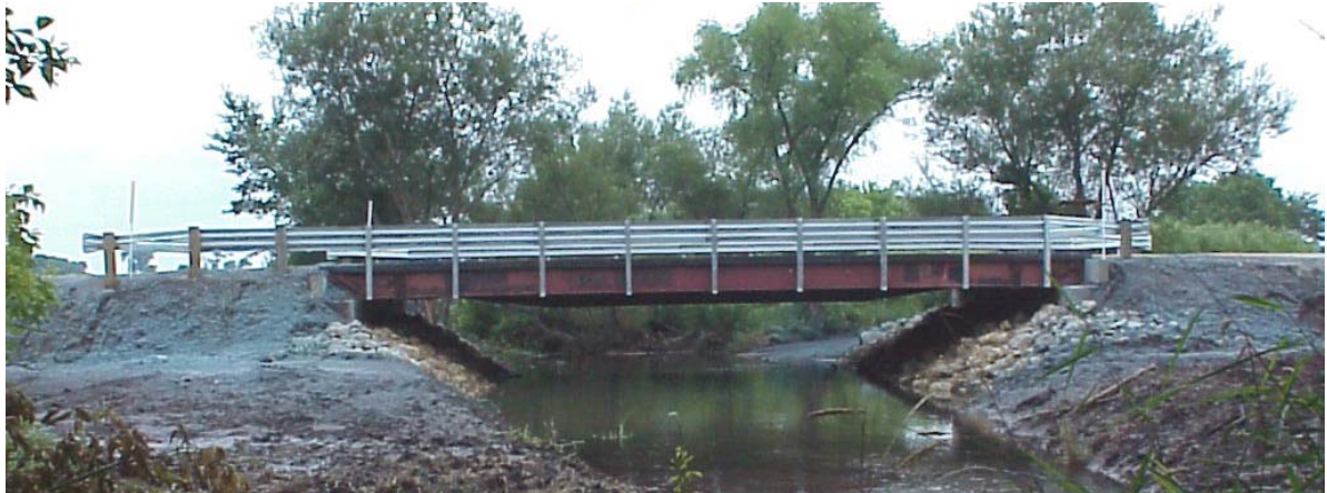
Figure 3.7. Finished Buchanan County RRFC Bridge.
