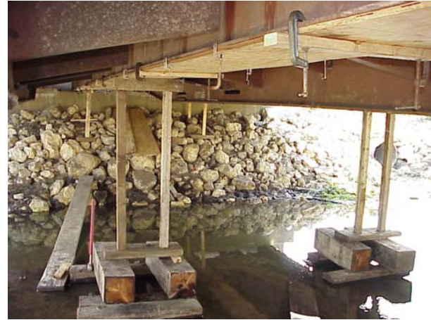
b. Formwork for concrete placement
