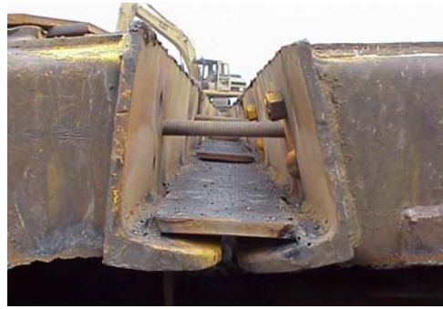
b. Bottom connection plates and threaded rod
