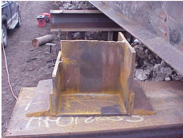
c. General shape of the exterior girder supports
