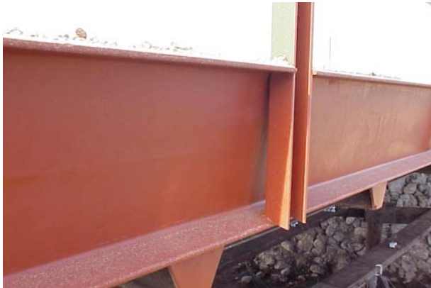
a. Addition of guardrail posts
