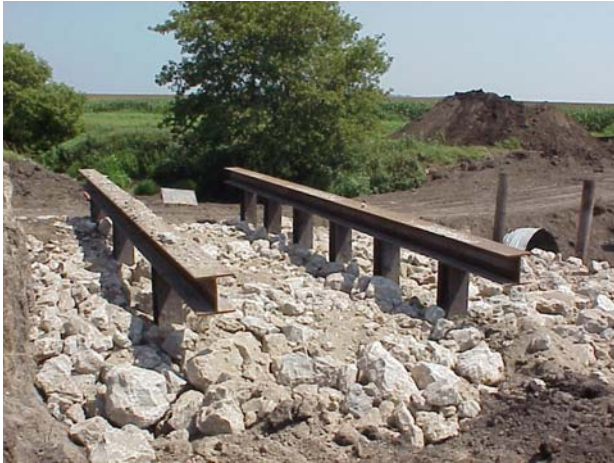
a. WCB north abutment and pier
