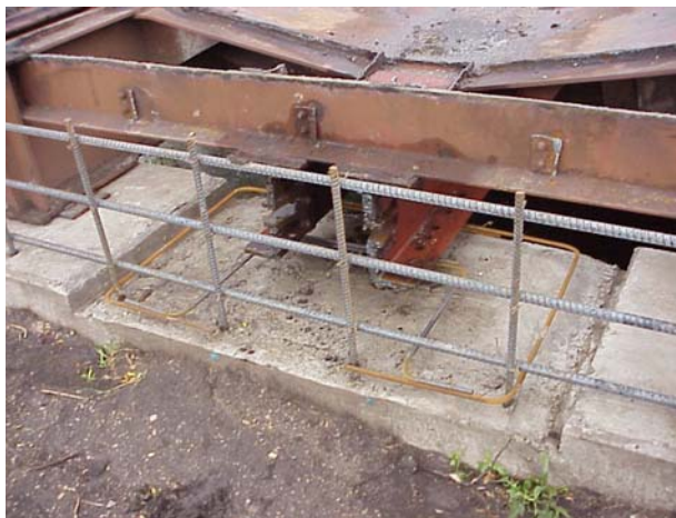
c. Backwall and interior girder seat reinforcement
