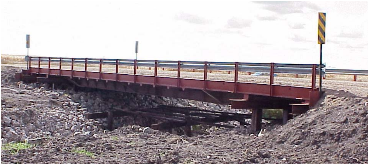
Figure 3.15. Finished Winnebago County RRFC Bridge.
