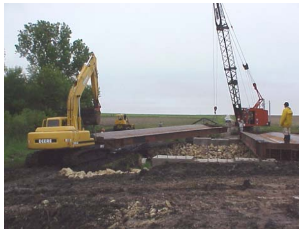
b. Flatcar placement on the cap beams
