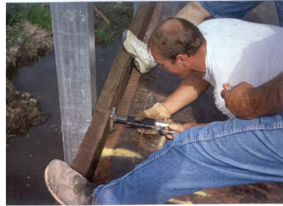
b. Nailing on the side rail for the driving surface
