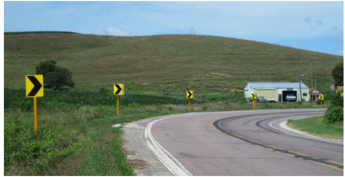
Figure 2. Additional delineation on existing chevron posts (Hallmark et al. 2012)
