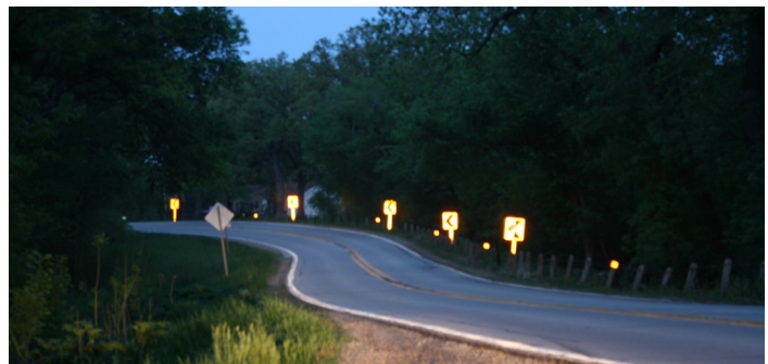
Figure 3. Reflective treatment added to existing chevron posts (Hallmark et al. 2012)
