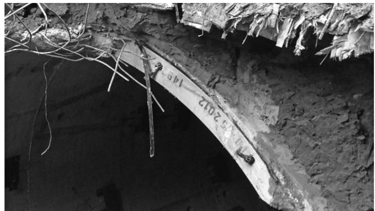
Fig. 4. View of the hardened grout as can be seen in the enlargement for a station. It is possible to observe how the mix fills completely the void annulus (photo Mapei's archive).
