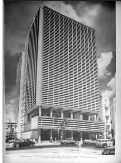
Retiro Odontológico building. Arquitectura , No. 282, January 1957, p.22-30
