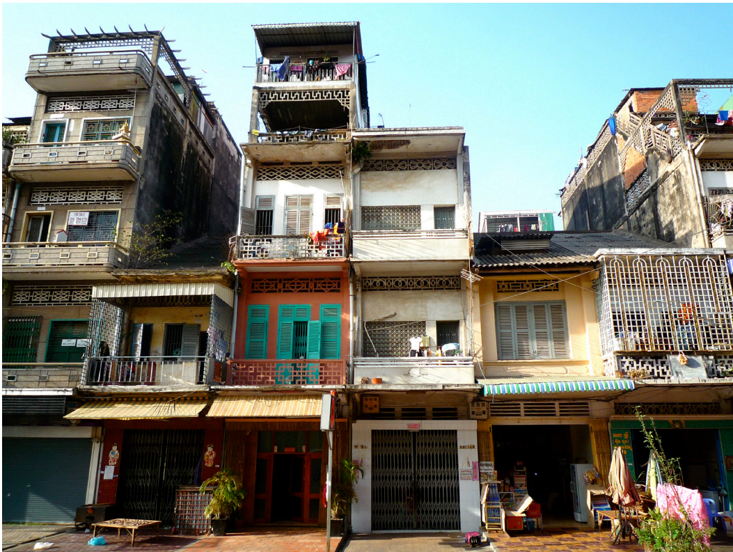
FIGURE 26: Shophouse design is extremely conducive to the incremental architecture building process. The widespread addition of floors to the existing, formal stock proves this compatibility. Photo by the author.
