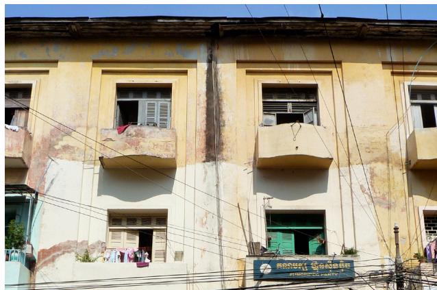
FIGURE 19: An art deco shophouse apartment building from the 1930s or 1940s. Thin, cantilevered horizontal fins shade the windows, a feature made possible by the use of reinforced concrete construction that was beginning to gain widespread use in the 1930s. Photo by the author.
