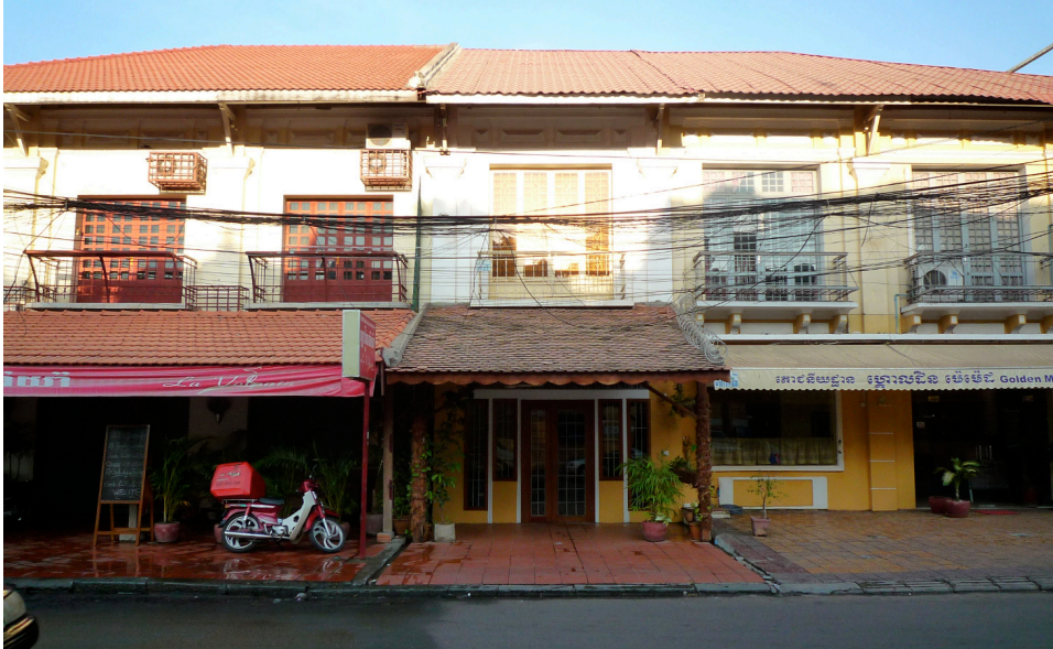
FIGURE 18: These two-story colonial, pitched-roof shophouses are representative of the permanent prototype which replaced its fire-prone counterpart at the turn of the 19th Century. Masonry foundations, brick walls, and tiled roofs ensured durability. Photo by the author.
