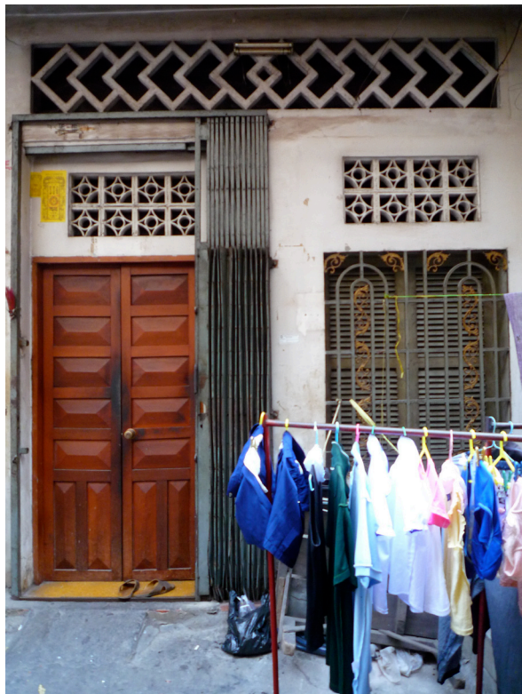
FIGURE 17: Decorative ventilation openings puncture shophouse façades, permitting natural light and air circulation. Pictured here is the back alley entrance of a mid- century shophouse. Photo by the author.
