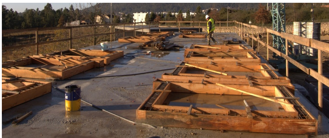
Figure 3.9 Wooden molds and reinforcement inside them
