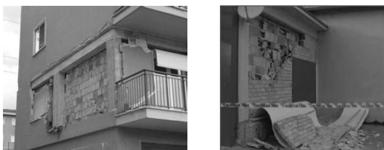
Figure 2.19 Detachment of the leaves in multi leaf walls [19]
