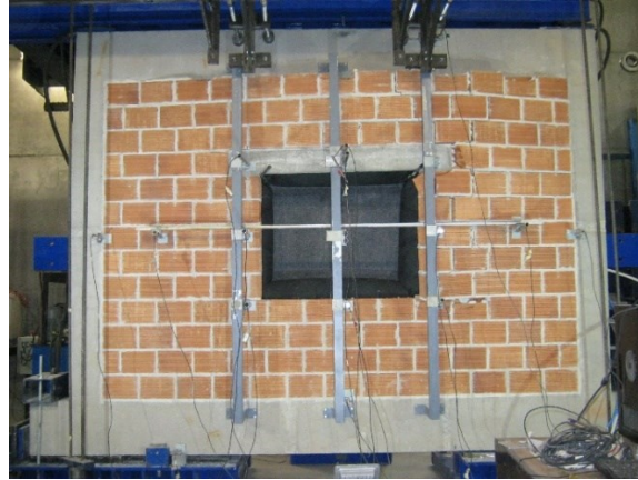
Figure 4.35 Out-of-plane failure of the right part of the masonry infill
