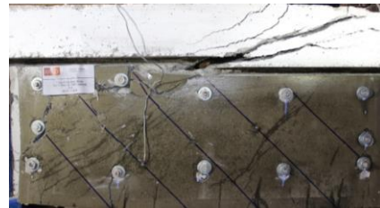
h) Final crack pattern of the T-5L45-B beam
