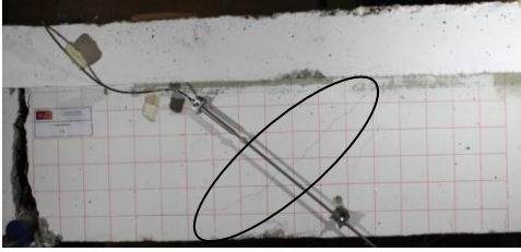
a) Crack pattern at failure load of T-C-R beam
