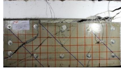
f) Final crack pattern of the T-3L45-B beam
