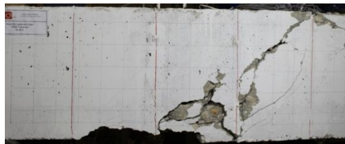
d) Crack pattern at failure load of the R-NSM-4L90 beam
