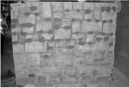
Figure 2. Construction of the semi-irregular masonry wall.
