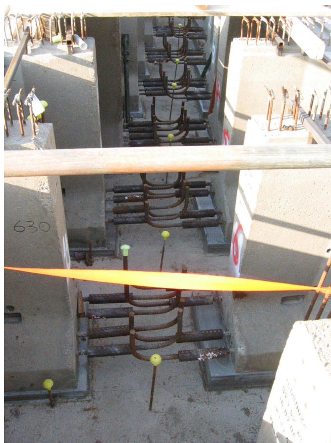
Fig. 5. (Color) Continuity of bridge beams (image by N. A. Hoult)
