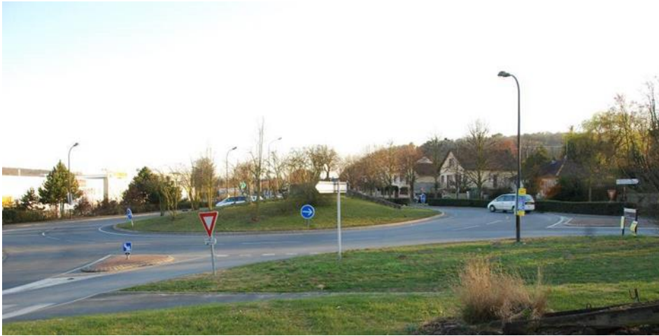
Fig. 27. A roundabout constructed on an outcrop of the ‘ Falun d’Etrechy ’, part of the historical Stampian stratotype, but nevertheless ignored by the local planning authorities (photo: P. De Wever)
