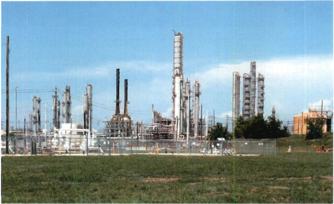
Vacant land owned by Exxon Mobil, Park Place subdivision
