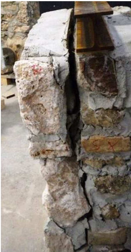
Fig. 7 Failure mode (unreinforced panel)
