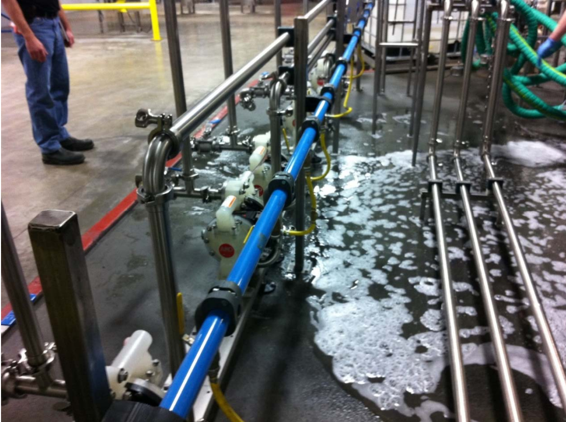
Figure 2-4: Diaphragm pump header regulated to 55 psig. Photograph by A.C. Harding, used with permission.
