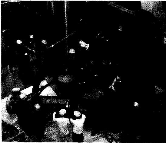
Fig. 4. Installation work of the full scale model at the experimental site.
