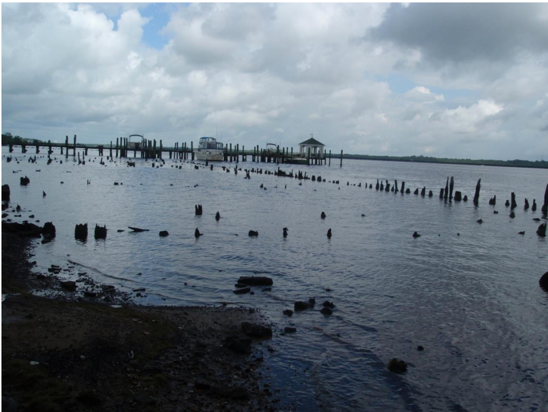
Figure A1.1. Photo of Kings Park beach and the northeast view of surviving pylons in the water (Photo 202 taken 5/16/2009 by Jeremy Eamick).
