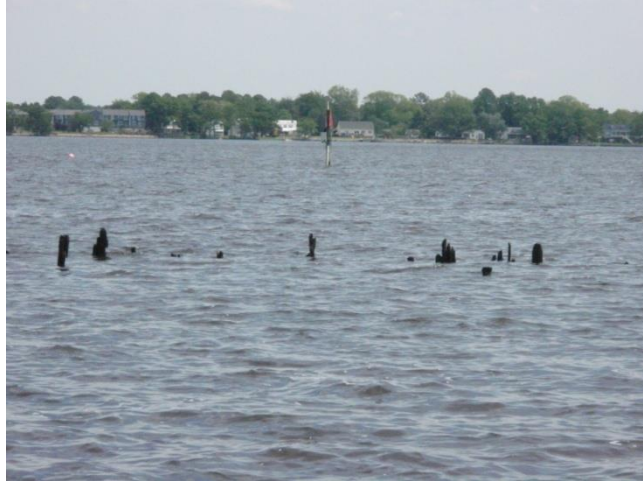
FIGURE 6.12. Photo of northern edge of pilings in the Neuse River. These pilings are located along King and Edgerton Street. These pilings are the remnants of the Neuse Lumber Co wharf, the southeastern corner (Photo130 taken 5/12/2008 by Jeremy Eamick).
