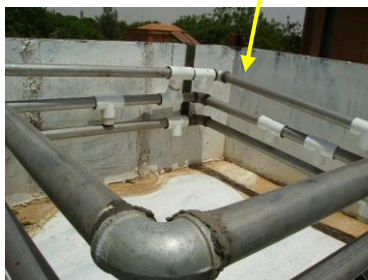
Fig.4.15 Condenser Coil in Tank
