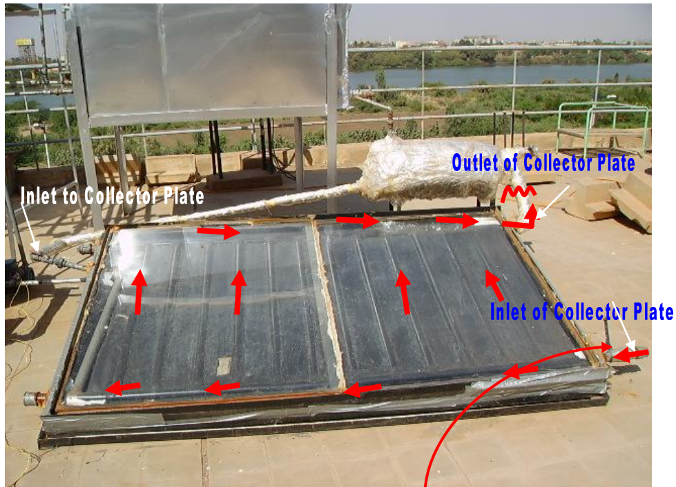
Fig. 4.34 Inlet and Outlet flow through the Collector Plate
