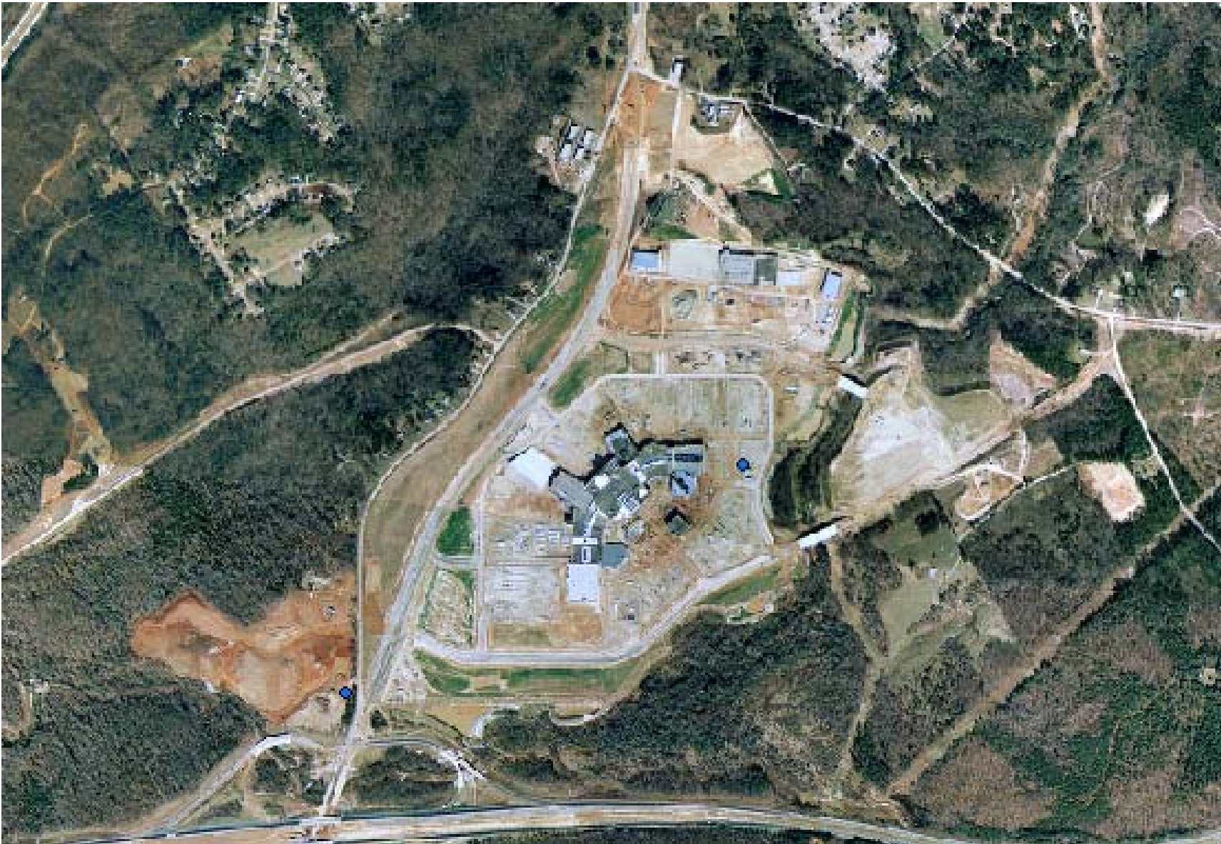
Figure 2.11. 1999 Aerials Express orthophotos. Example showing the Mall of Georgia during construction.
