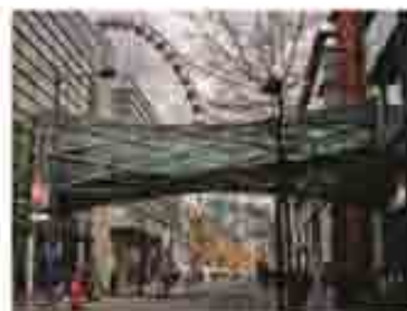
Figura 143 – Ponte sobre a Corporation Street (Manchester)
