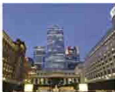
Figura 205 – Cabot Hall / Cabot Square, Canary Wharf (Londres)
