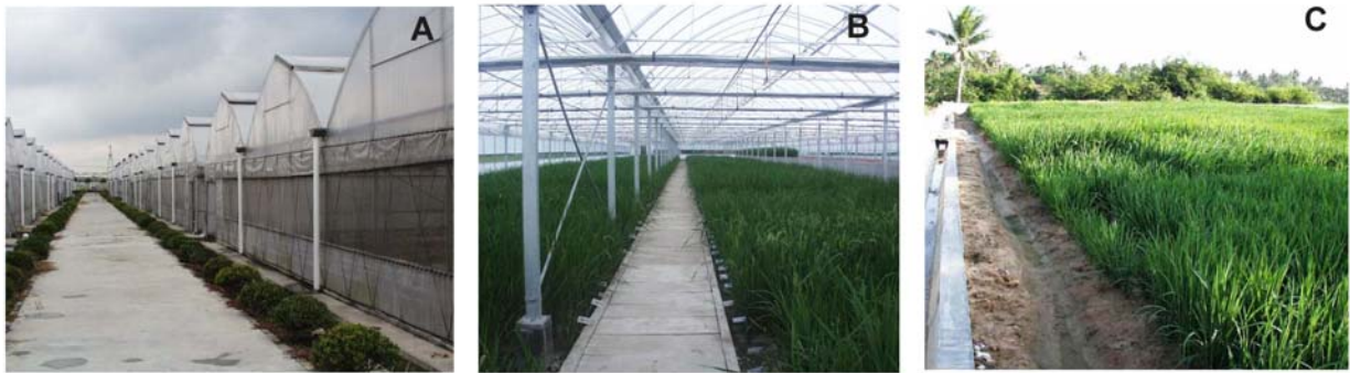
Figure 2. In 2001 and 2002 the Shanghai Agrobiological Gene Center-Shanghai Agriculture Academy of Science constructed over 2000 sq meters of specialized plastic greenhouses (A&B). The facilities include overhead sprinkler and surface drip irrigation capacity, deep (1.8m) drainage systems, and air ventilation capacity. Early experience illustrates the importance of managing the “microclimate” over the crop to simulate realistic field level evapotranspiration as well as the soil water status. C. Field screening facilities on Hainan Island allow large scale off-season (winter-spring) field screening for drought tolerance.
