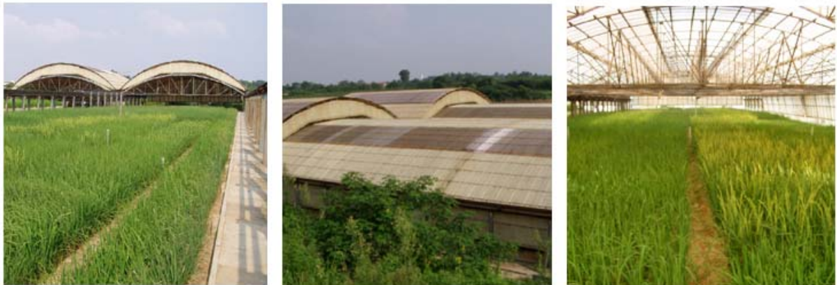
Figure 3. Researchers at the National Key Laboratory of Crop Genetic Improvement, Huazhong Agriculture University, Wuhan, China have constructed perhaps the world’s first large scale “rainout shelter”. This facility assures control of the water regime to field screen rice for drought tolerance. The structure has an experimental area of 1,800 sq meters and incorporates rain sensors to close the double-layer roof thus protecting experiments. Unlike rainout shelters for other crop species, this structure incorporates deep soil and ground water table management and drainage (2.0 m deep concrete valved-drains) and surface and sprinkler irrigation facilities to simulate water deficits under large-scale rice cultivation.
