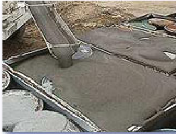
Figure G3-2. Filling voids around drums at EnergySolutions Facility in Utah. Figure copied from EnergySolutions Web site.
