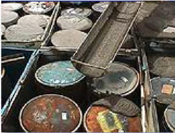
Figure G3-2. Filling voids around drums at EnergySolutions Facility in Utah. Figure copied from EnergySolutions Web site.
