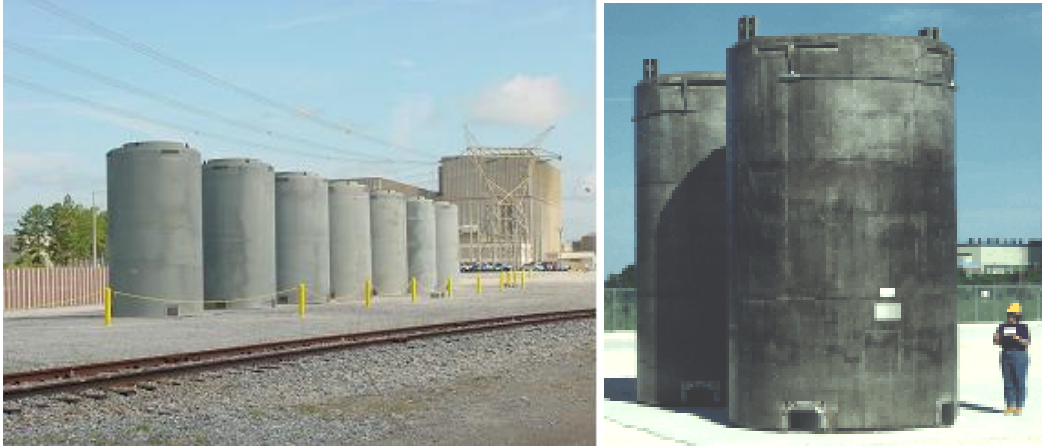
Figure E2-8. Typical dry storage casks.
