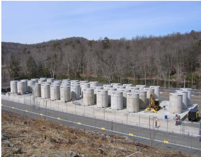
Figure E2-9. Overview of typical dry storage pad.
