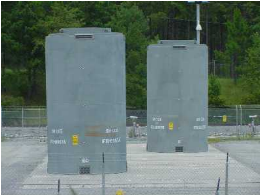
Figure G2-3. Holtec International HI-STORM Dry Storage Casks on storage pad (note vertical storage). Figure copied from Holtec International Web site.
