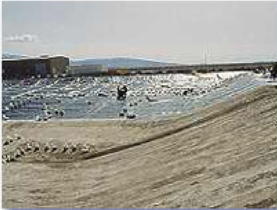
Figure G3-4. Landfill disposal cell at EnergySolutions (Note line and leachate collection piping). Figure copied from EnergySolutions Web site.
