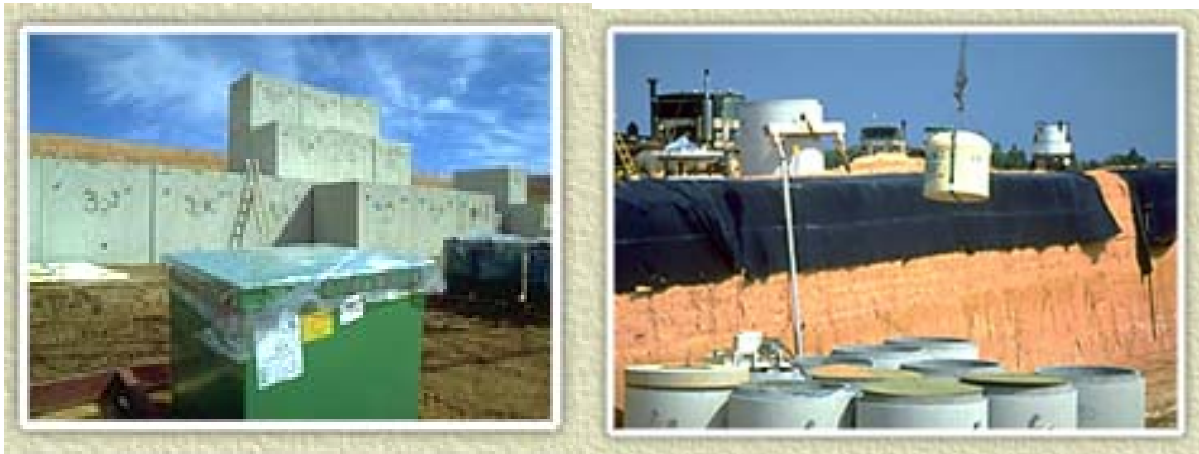
Figure G3-5. Waste placement in landfill at Chem-Nuclear Systems Barnwell site. 11
