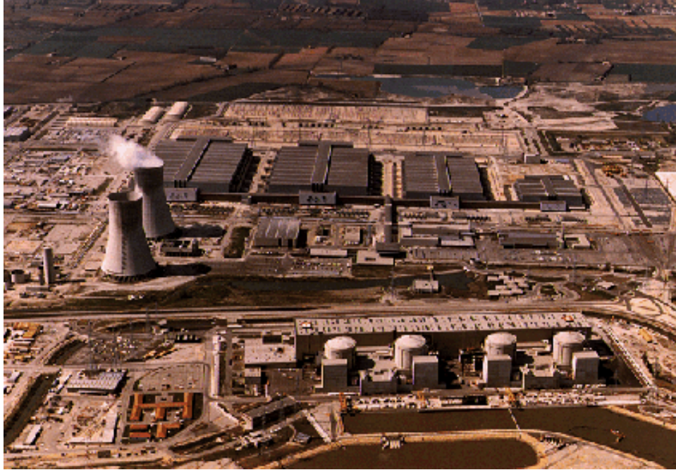
Figure C1-6. George Besse Gaseous Diffusion Enrichment Plant.
