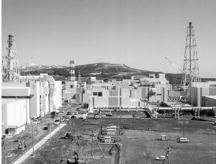
Figure F1-4. Rokkasho-Mura site, Japan, with Rokkasho Reprocessing Plant (JNFL).
