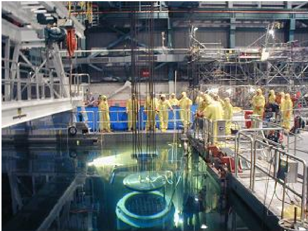
Figure E2-5. Cask for dry fuel storage being closed under water for shielding protection.
