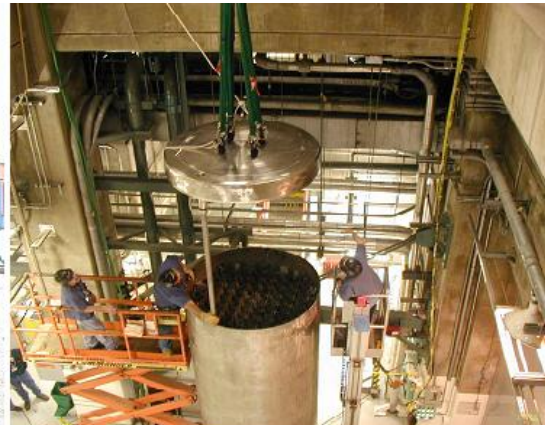
Fit up of the MPC and MPC Lid at J.A. FitzPatrick Nuclear Plant
