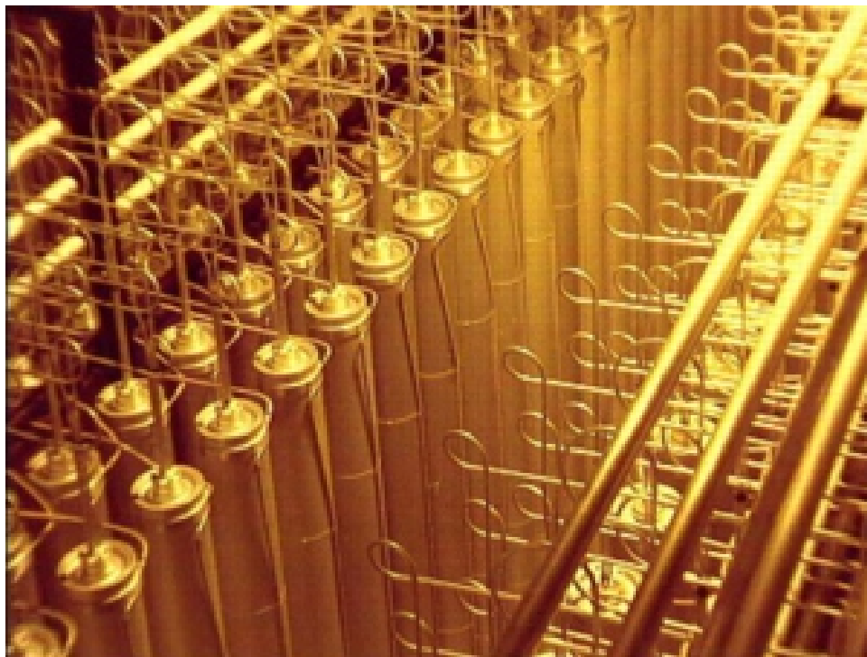
Figure C1-9. Top view of a bank of centrifuges at a URENCO gas centrifuge plant.
