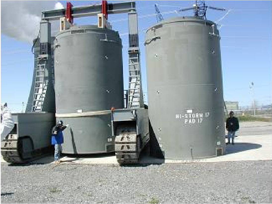
Figure E2-6. Cask being placed on dry storage pad.
