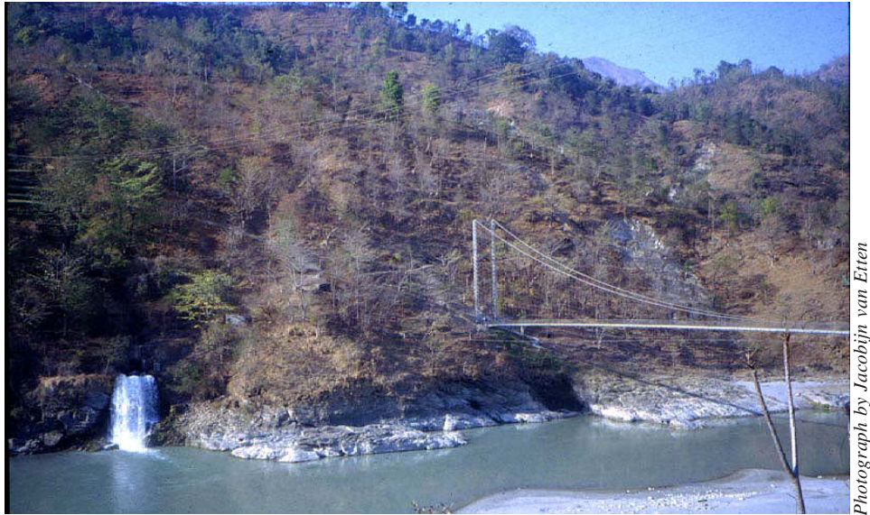
Figure 1. Siphoning of water from the main irrigation scheme to the Asardi sub-scheme in the Andhi Khola Irrigation Scheme.
