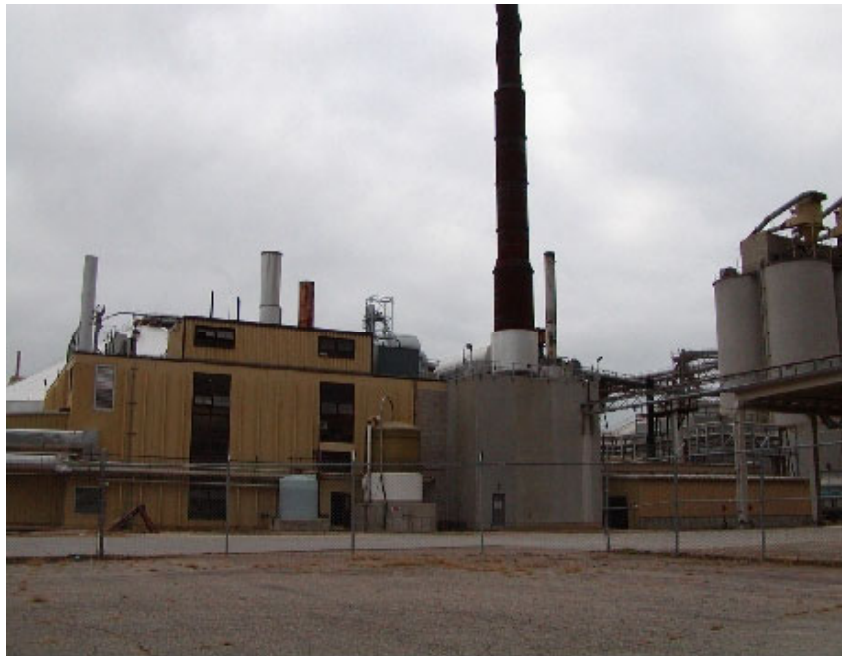
Figure 7. Mankato, Minnesota, Crushing Plant
