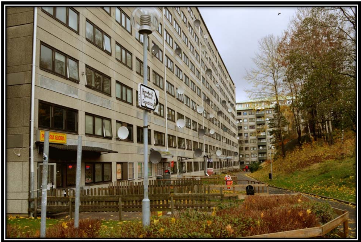
Figure 2 Bredfällsgatan, where the 85 apartments in the case study are located (Photo: Frederick Nyandiko).
