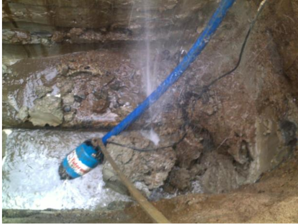
Figure 5 Grey cast iron pipe failure Type A (left), easily repaired with a repair clamp (right). Photo Annika Malm.
