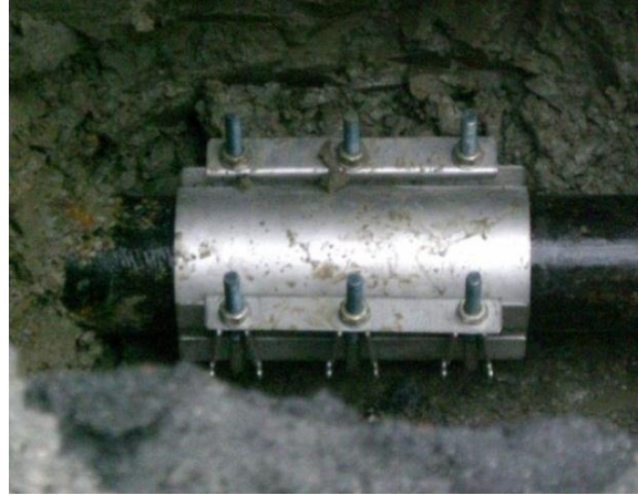
Figure 5 Grey cast iron pipe failure Type A (left), easily repaired with a repair clamp (right). Photo Annika Malm.
