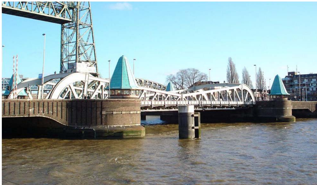
Figure 1 Koninginne Bridge Rotterdam
