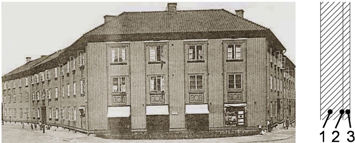
Figure 3. Landshövdingehuset “County governor’s house” in Gothenburg, Sweden. A façade in 1930 (left) and the construction of the original wood wall (right). 1) Structural wood or brick, 2) Tar paper, 3) Wooden cover boarding. (Photo from Sören Nilsson’s collection of postcards; Pär Johansson).
