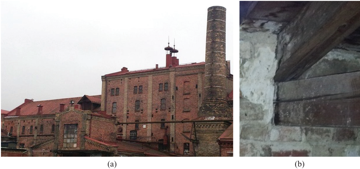
Figure 1 (a) An old industrial building considered to have a façade with special aesthetic values that should be preserved and (b) a connection between a wooden beam and brick wall.
