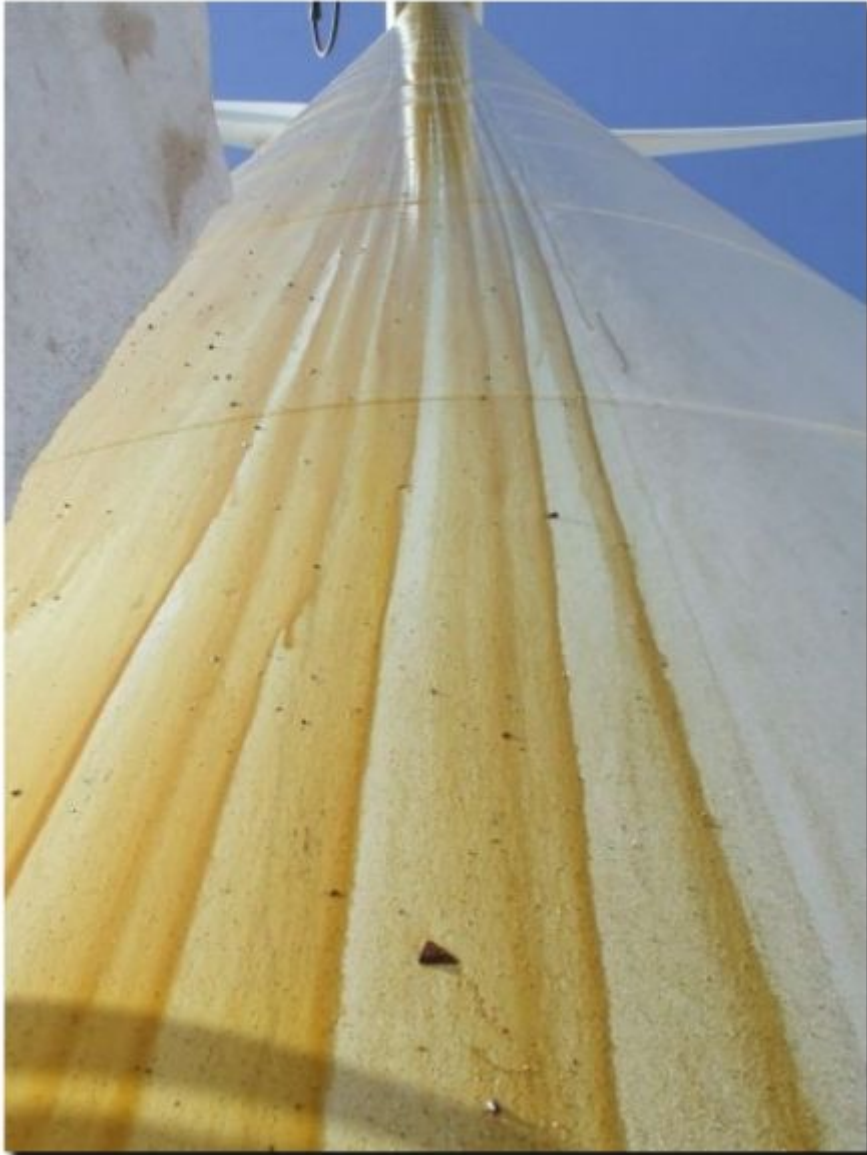
Photo of oil leakage from wind power plant. Source: http://www.iberica2000.org/documents/eolica/photos/contamination/ .
