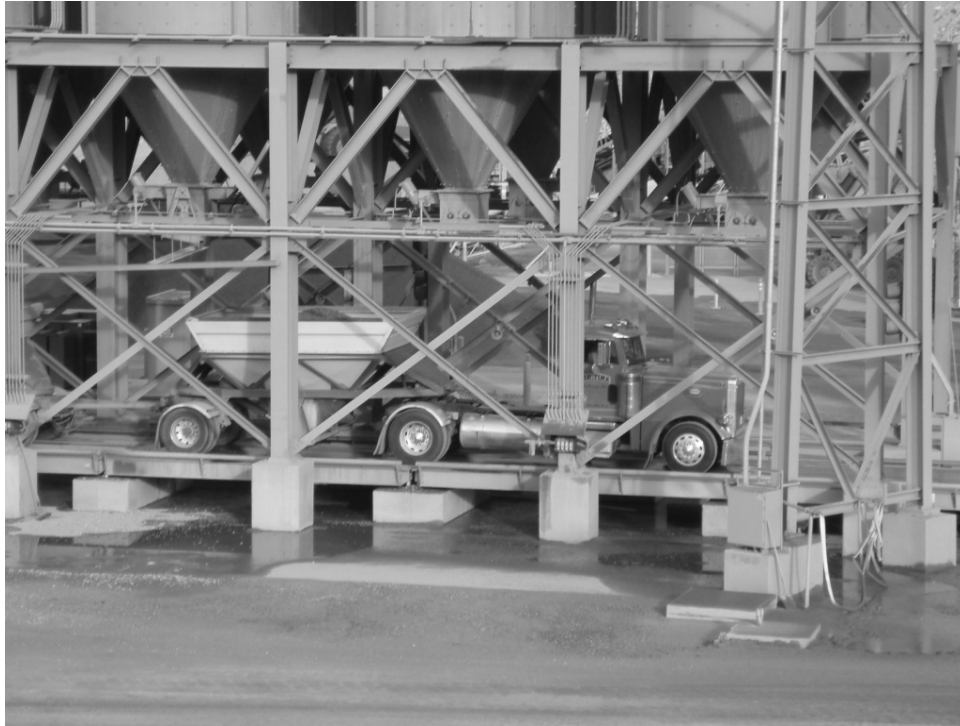
Figure 3. Loading and weigh station at the same place. VMC's Reliance operation, Irwindale, CA, USA.
