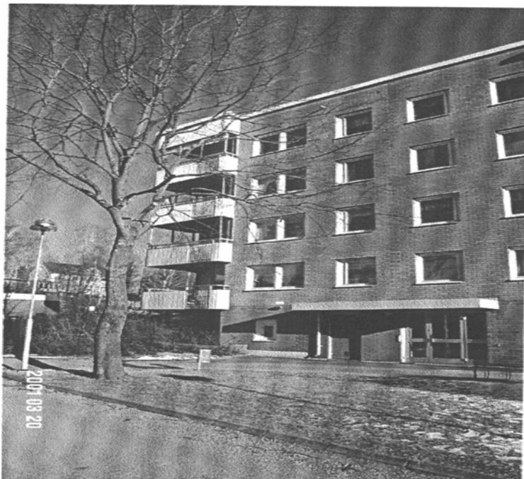
Figure A7.1. Facade of the test building, facing towards NW. The length axis of the building is orientated SW-NE.
