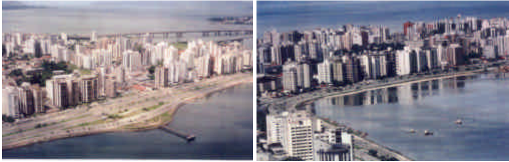
Fig. 16 – Aerial photographs of the new modern residential areas in the North Bay. Source: Alina G. Santiago.
