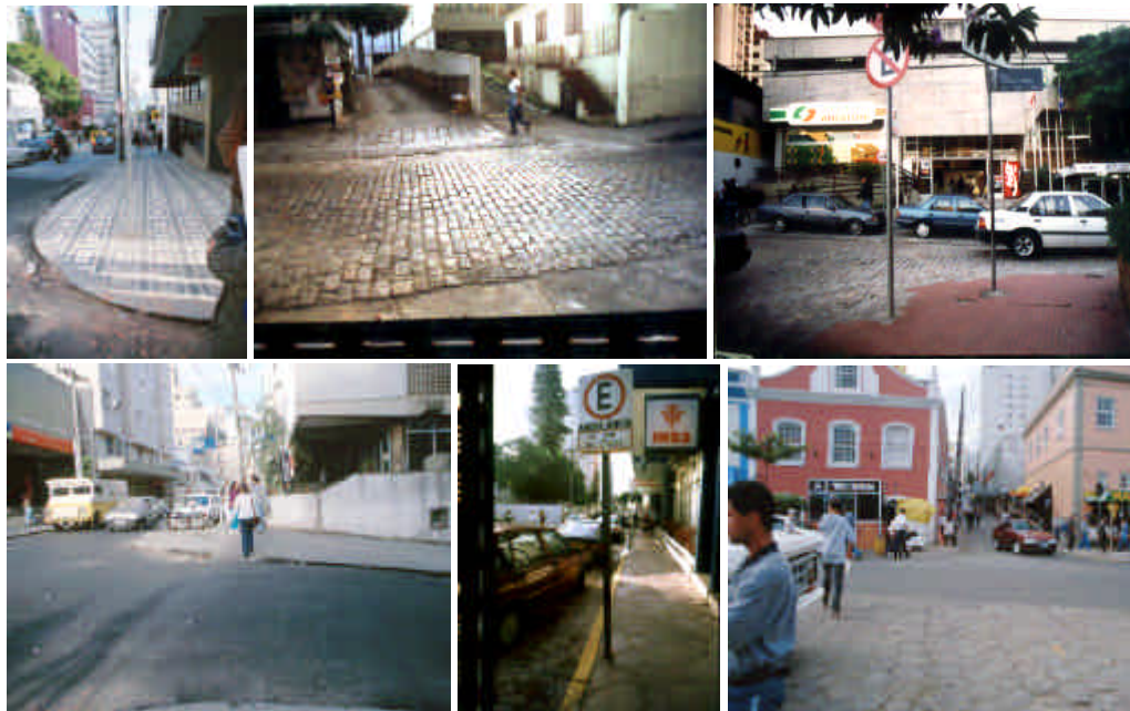
Fig. 42 – Illustration of the different problems: declivity (1), irregular limits of the pathways (2), visual pollution and excess of obstacles (3), lack of information and access to public services (4, 5) and dangerous crossings (6).
