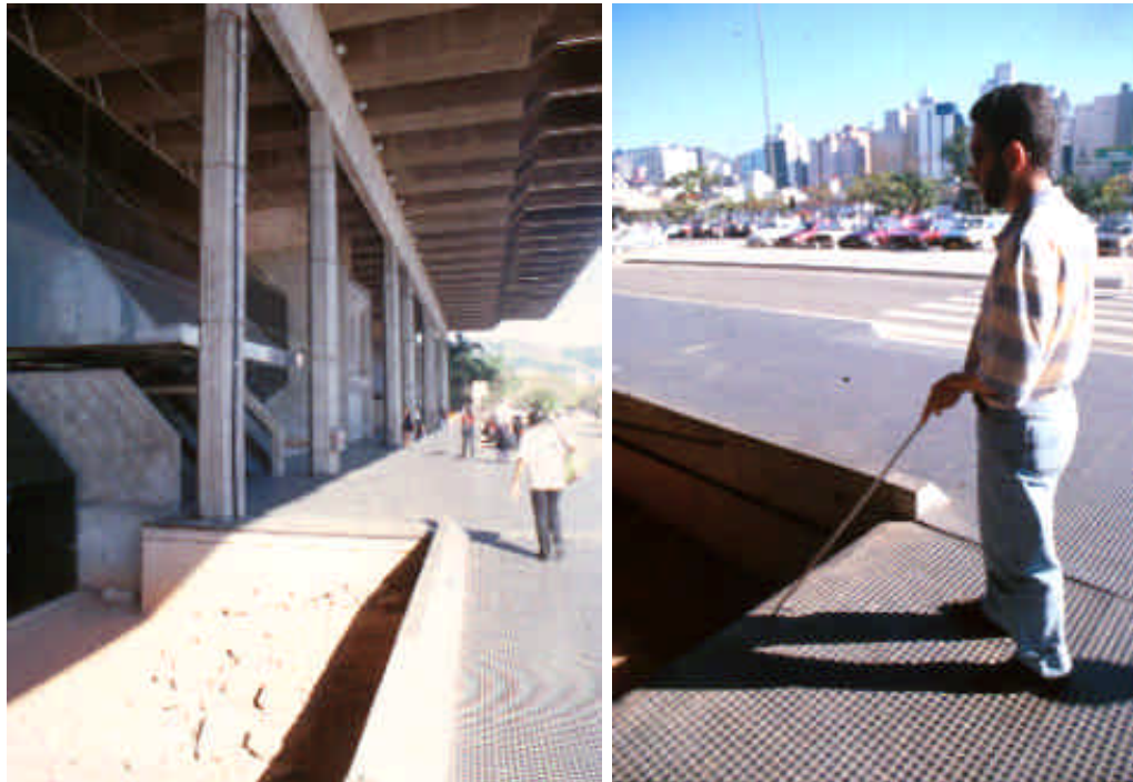
Fig. 33 – Photographs taken in the interstate bus station during the first ‘Accompanied Walk’. On the left photograph can be seen the wide pathway with no marking of the entrances, on the right picture, the ditch without protection.
