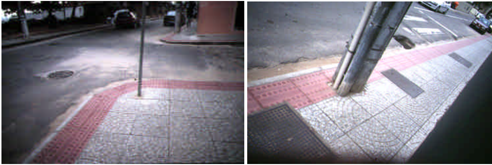
Fig. 49 – The impossibility of removing the electricity poles, and the careless in replacing traffic-posts turned the borderline pavement meaningless. In some parts it can be observed that the excessive texture of the barrier-free pavement makes more difficult the recognition of textures contrast.
