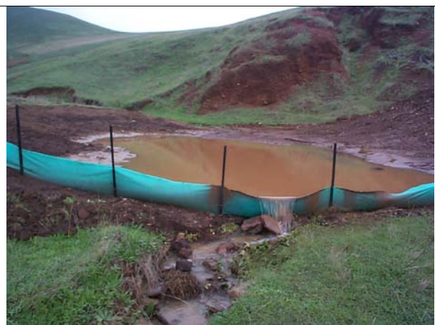
Silt Fence Sediment Trap
