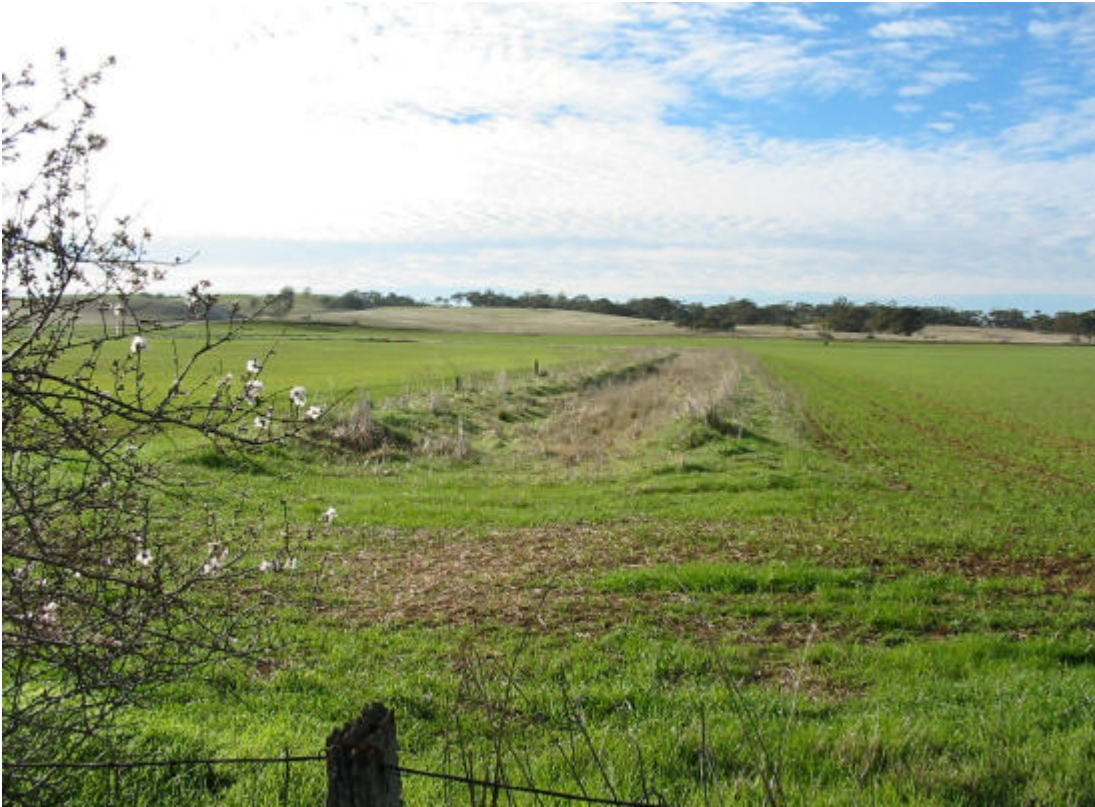
Excavated from floodout area at base of hill slope to a roadside table-drain
