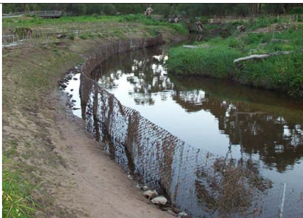
Alignment Fencing After Construction
