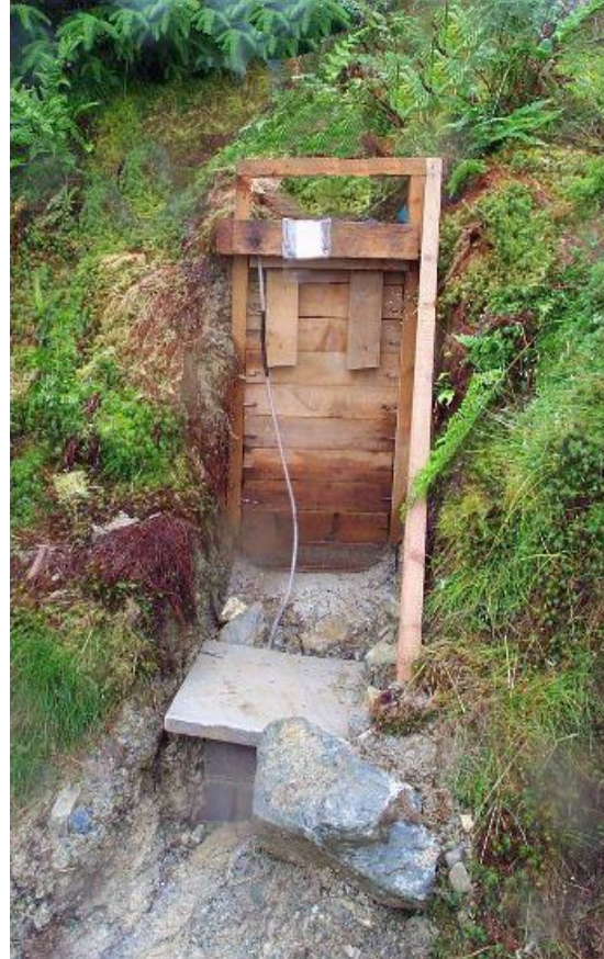
Figure 6(b) Site after installation of water flow recorders and data loggers
