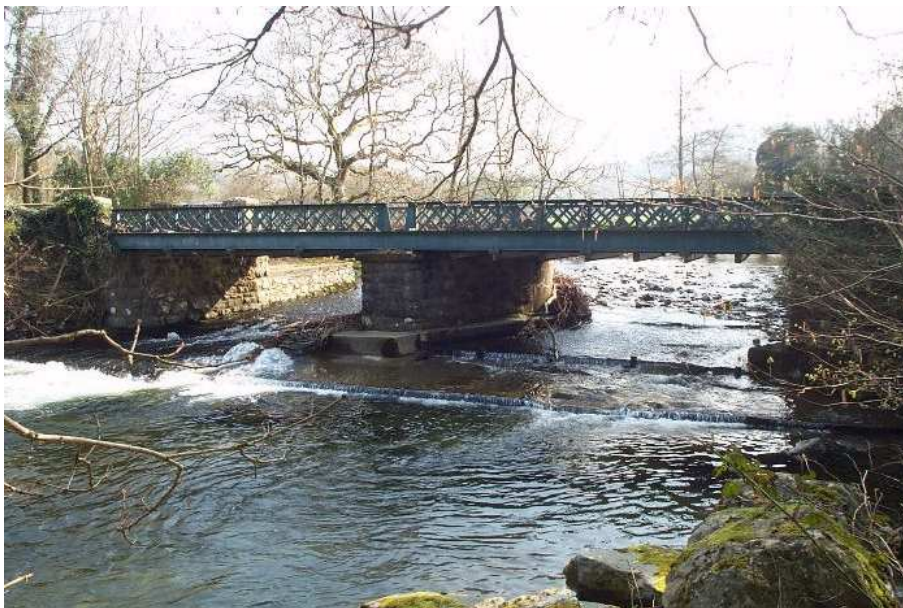
Figure 25 : Weir at Dolserau bridge
