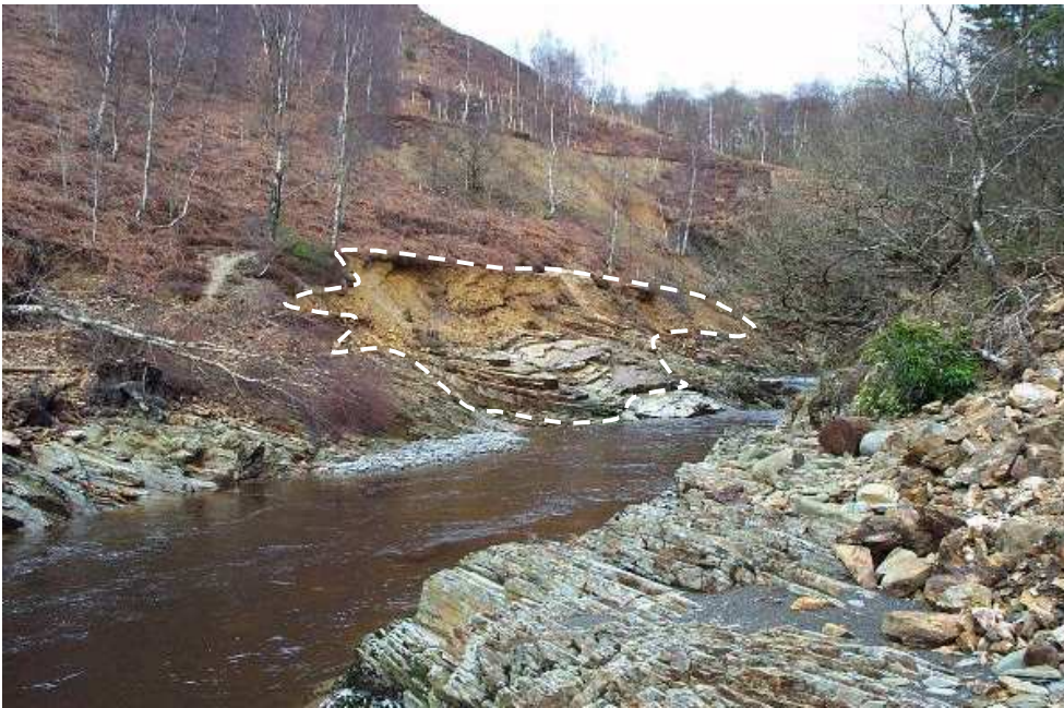
Figure 18(a): Zone of sediment loss during the July 2001 flood event. Afon Mawddach at Bedd y Coedwr.
