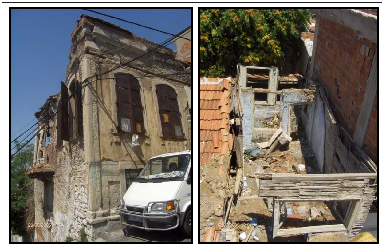
Photo 2: Ruined Historical Buildings
