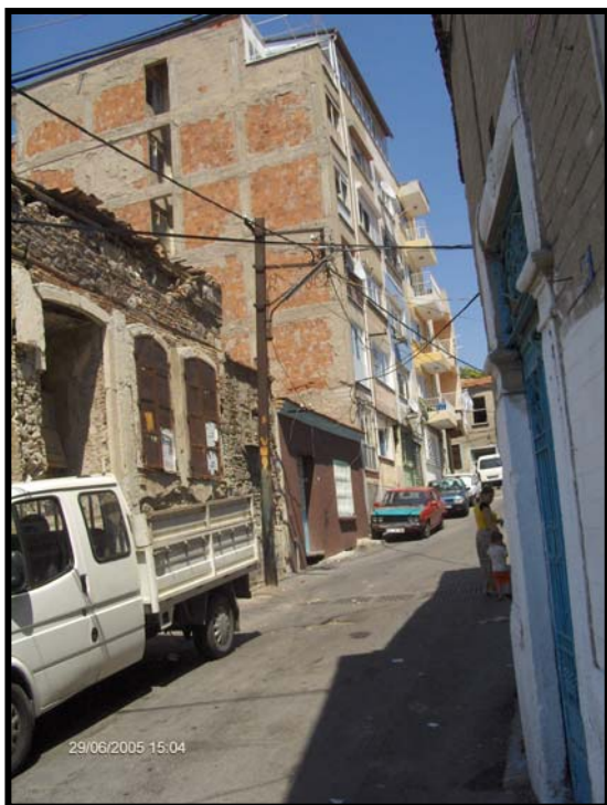
Photo 1: Some of the Illegal Buildings in the Area
