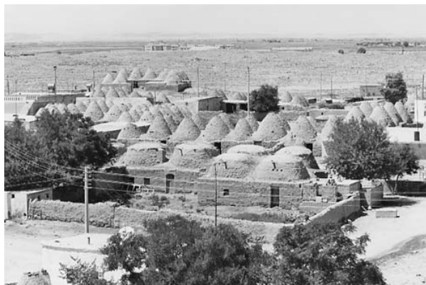
Photo 2 . Traditional Harran Houses
