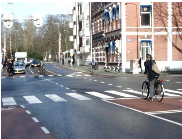
Figure 1.2: Bicyclists have a separate waiting area in front of cars at a major intersection in the city of Groningen in the Netherlands.
