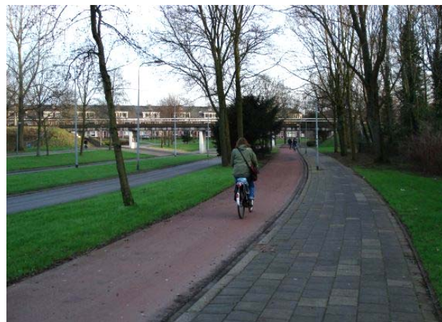
Figure 1.3: A bicycle lane going towards town turns into a separate path and stays flat as it and the roadway go under a bridge.
