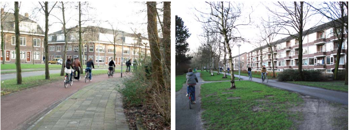
Figure 2.1: Bicycle paths separate from the roadway consistently found to be most preferred bicycle facility in stated-preference surveys.
