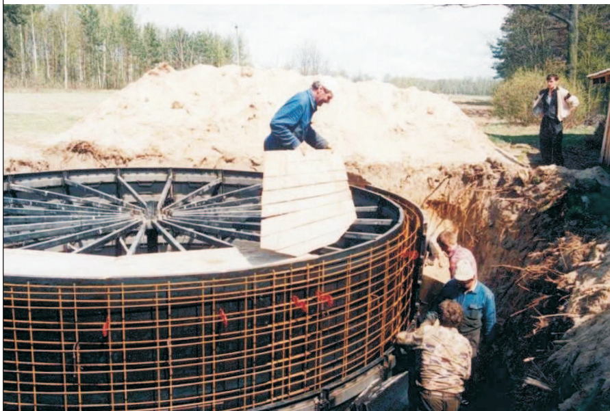
Figure 2: Construction of Slurry Storage Tank in Poland
