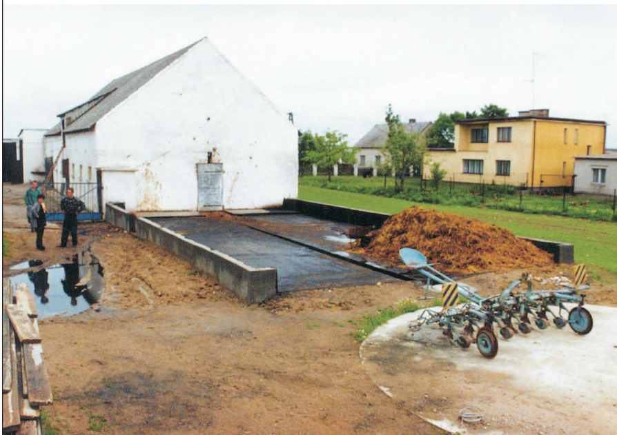
Figure 5: Manure Stored on Concrete Pad
